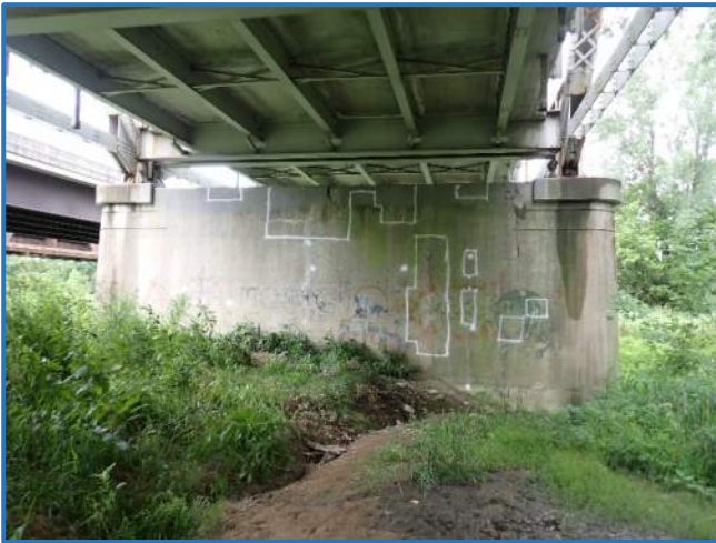
Photo 82 - East face of Pier 4
