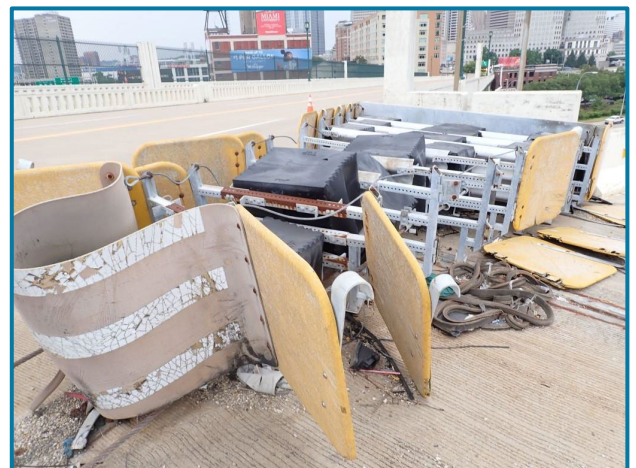
Photo 12 – Damaged crash attenuator with hanging panels, deployed cushions, and loose cables (looking west).
