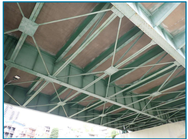
Photo 24 – Approach span girders (Span 14 shown, looking south).
