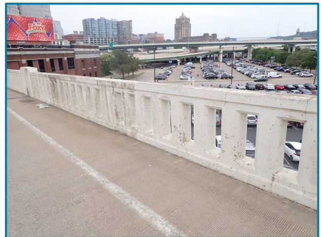
Photo 7 – Bridge railing (looking northwest).
