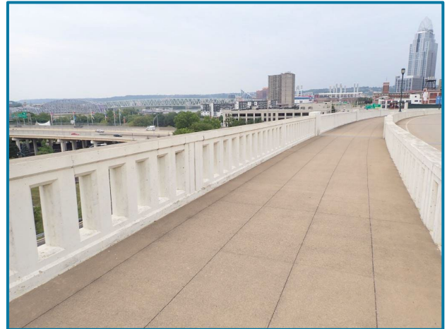
Photo 23 – Pedestrian sidewalk on the south side of the bridge (looking west).
