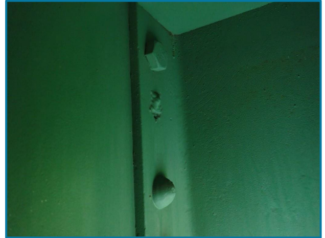
Photo 56 – Rivet head has been torch cut off (U20 of the North Truss, Span 11).
