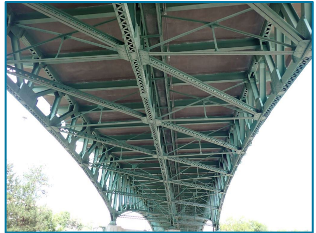
Photo 32 – Steel truss has three truss lines (Span 6 shown, looking east).
