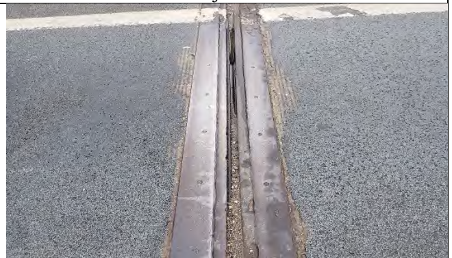
Photograph 16: View of the sunken joint seal over Pier 2 on the south end.
