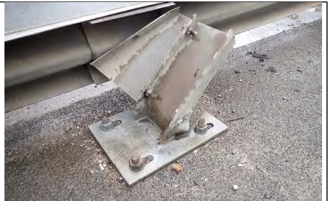
Photograph 20: Impact damage to the first post for right rear rail, Span 1, looking northeast. No change.
