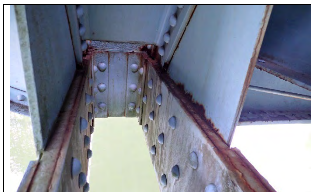
Photograph 45: Typical example of pitting along the lower chord gusset plate interior face shear plane. L2 rear left truss shown looking east.
