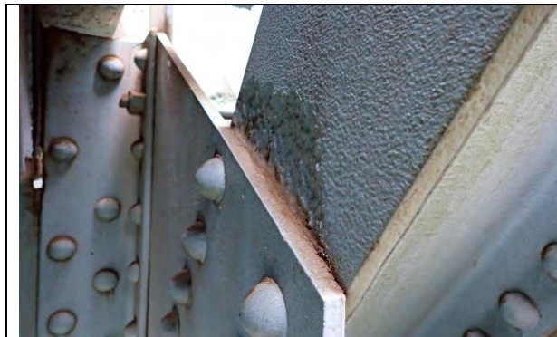
Photograph 32: View of typical painted over pitting on truss diagonals at lower gusset plates. U2L3 right truss shown looking southeast.
