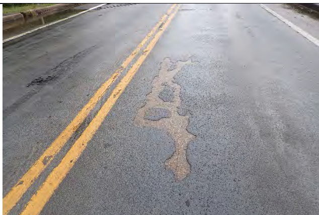
Photograph 8: Larger than normal example of wear occurring on top of the wearing surface in Span 4 eastbound.
