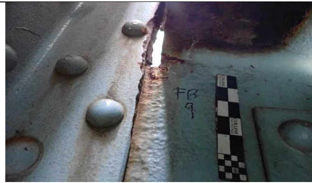
Photograph 37: View of cracks at Floor Beam 9 left (north) truss. Overall view looking east.
