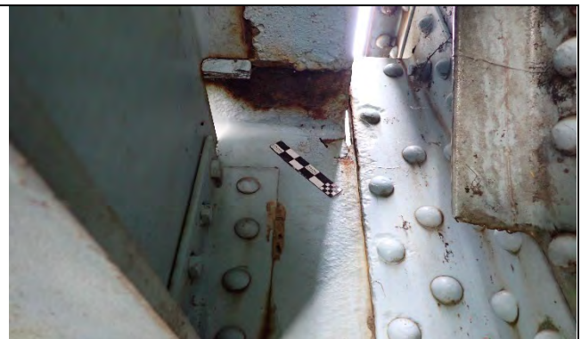
Photograph 34: View of cracks at Floor Beam 0 left cope. Overall view of detail.
