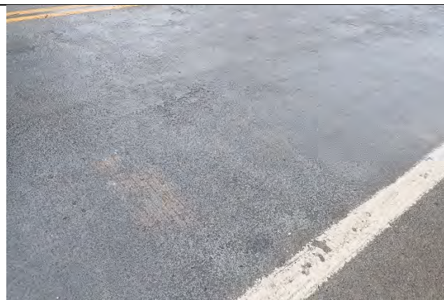
Photograph 7: General example of wear on the overlay, Span 1 near Pier 1 shown.
