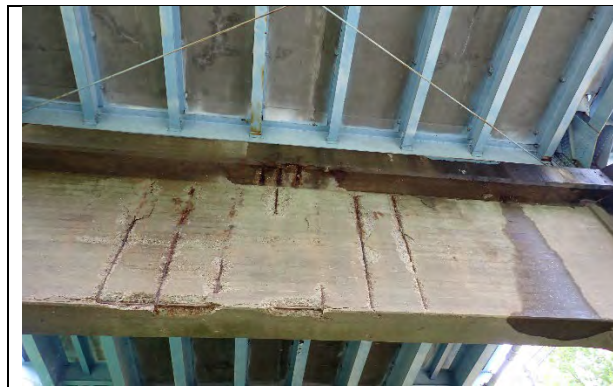
Photograph 54: Overall view of the rear face of Pier 2. Note extensive spalls and exposed reinforcing steel.
