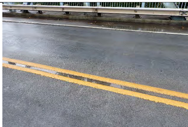
Photograph 6: Typical example of transverse and longitudinal cracks on the wearing surface. Span 2 eastbound near Pier 1 shown.
