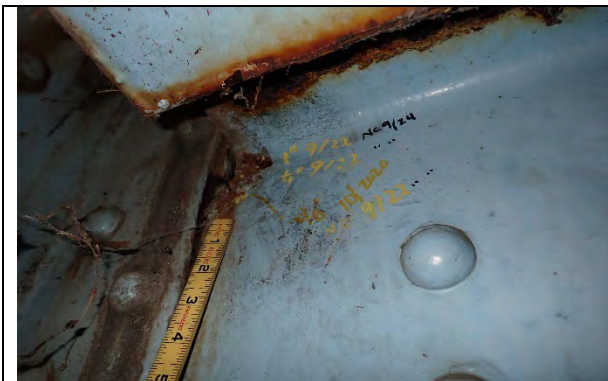
Photograph 33: General view, Floor Beam 9 right (south) truss cracks
