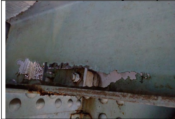
Photograph 27: General example of corrosion hole on the bottom of the sidewalk stringer web, Span 2.
