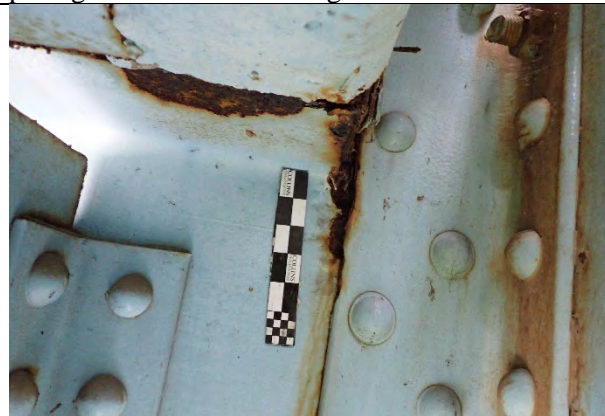
Photograph 43: Typical example of floor beam web pitting near the truss connection.
