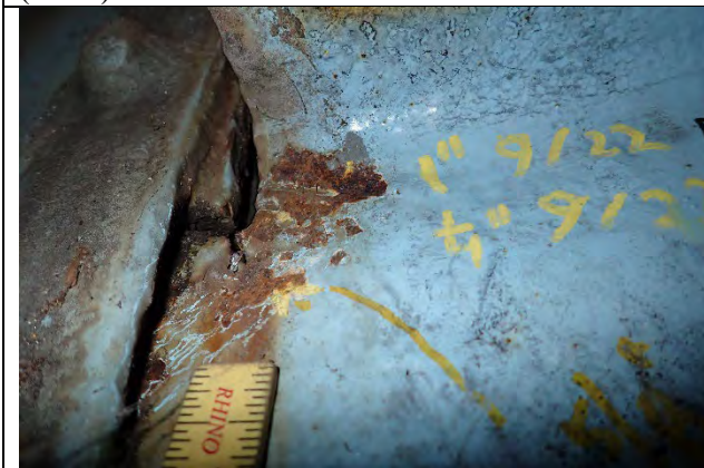
Photograph 35: Close up view, Floor Beam 9 right (south) truss cracks
