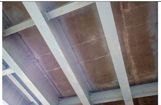
Photograph 4: General example of transverse and map cracks with efflorescence on the soffit. Span 1 between Girders 4 and 5 shown.
