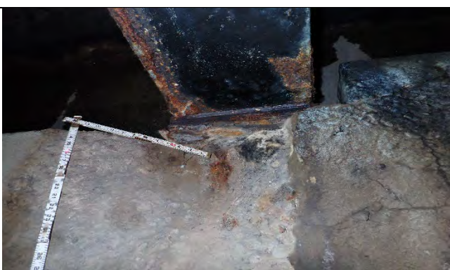
Photograph 51: Forward face of Pier 3, under Beam 4. Note no major change to spall undermining the bearing up to 5-1/2".
