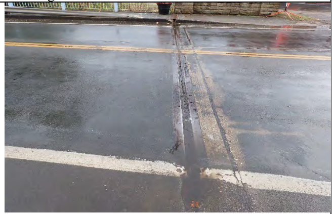
Photograph 14: Overall Rear Abutment joint, looking south. Note debris in the joint.
