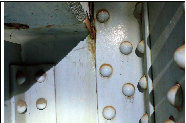
Photograph 40: Typical example of pitting on the floor beam web at truss floor beam connections.
