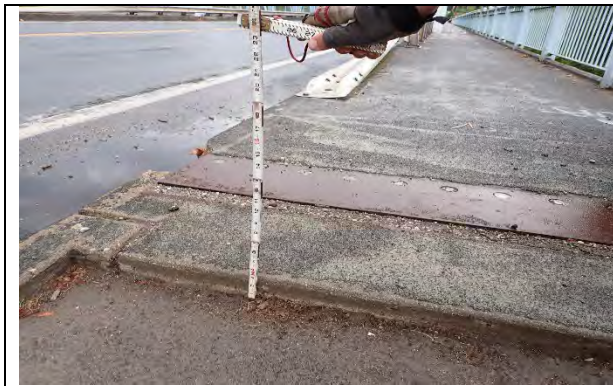
Photograph 60: View of the settlement to the rear right (southwest) approach sidewalk.
