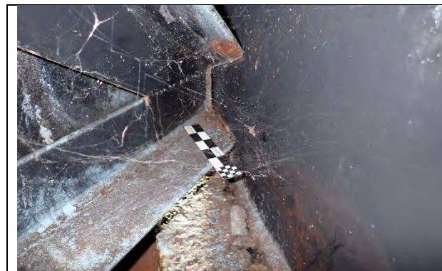
Photograph 23: Beam 4 at the Forward Abutment, north face. Note no change to broken cross frame weld.
