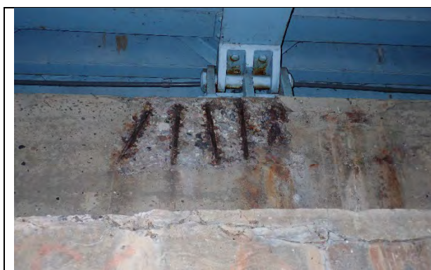
Photograph 50: Rear face of Pier 3 under Beam 6. Note no change to spall under the beam.
