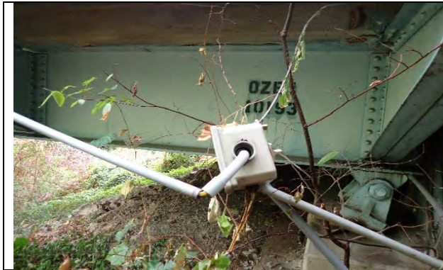
Photograph 57: No change to the broken conduit at the north side of the bridge near the Rear Abutment.
