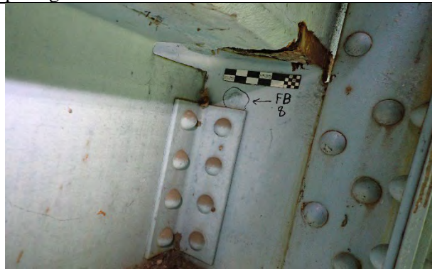
Photograph 42: Typical example of floor beam web pitting near the truss connection.
