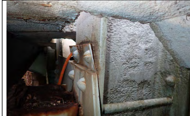
Photograph 31: Typical example of painted over pitting on truss vertical webs at the sidewalk level above lower panel points, L2 right truss shown looking southeast.
