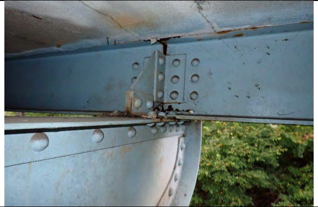
Photograph 28: typical configuration of sidewalk stringer and cantilever.
