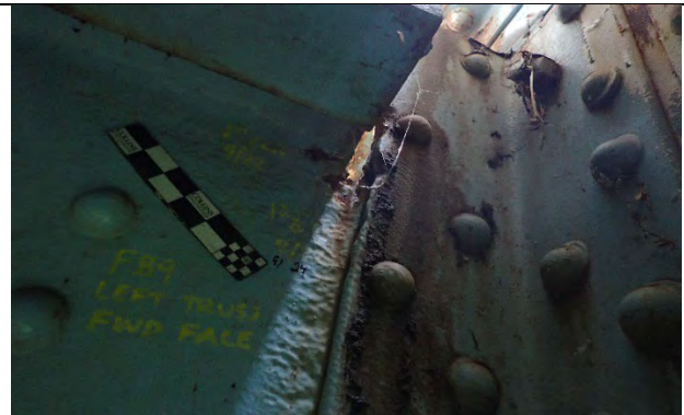
Photograph 38: View of cracks at Floor Beam 9 left (north) truss. Overall view looking east
