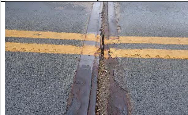
Photograph 15: Close up view of the Pier 2 joint near the centerline. Note the hole in the joint seal.
