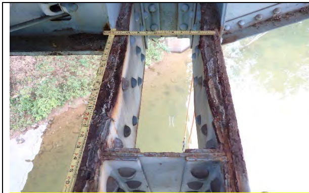
Photograph 30: View of pack rust on L6L7 right truss. Looking east.
