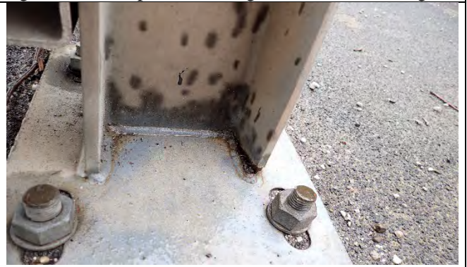
Photograph 22: Impact damage to second post for the right rear rail, Span 1, looking east. No change.
