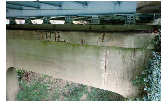
Photograph 54: Overall view of the rear face of Pier 2. Note extensive spalls and exposed reinforcing steel.
