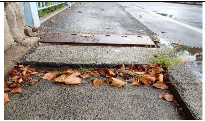
Photograph 61: View of the settlement to the rear left (northwest) approach sidewalk.
