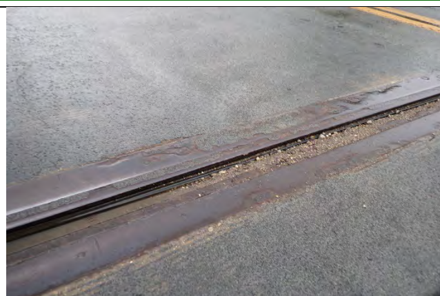
Photograph 18: View of the Pier 2 vertical offset and snowplow damage. Looking southeast.
