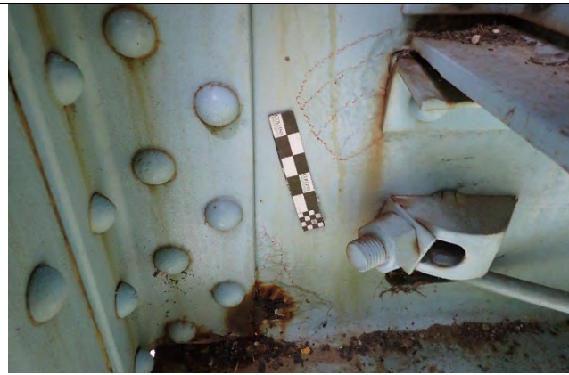
Photograph 44: Typical example of floor beam web pitting around the end stringer connection.
