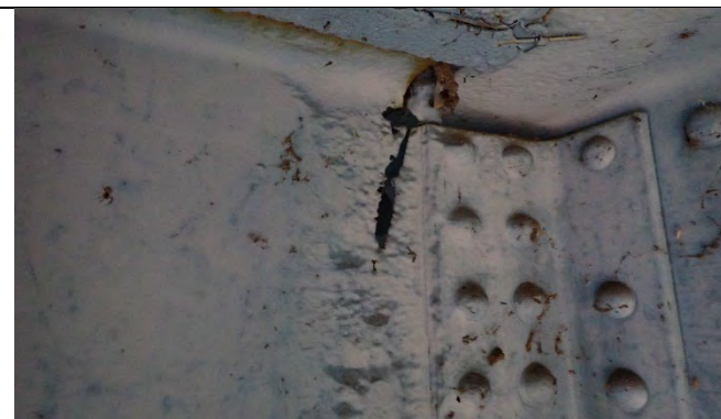
Photograph 24: View of corrosion hole on diaphragm between Beams 1 and 2 at Pier 3 Span 3. Looking west.
