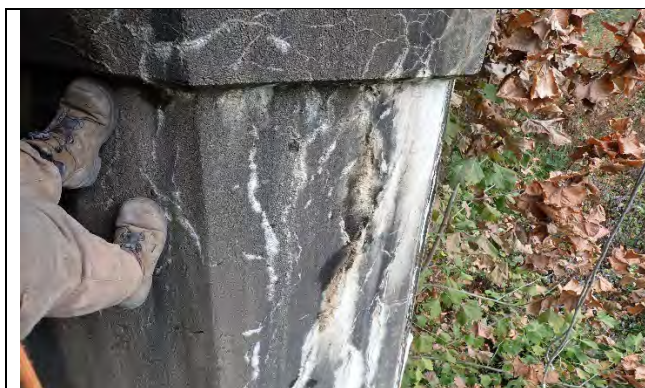
Photograph 49: View of the heavy efflorescence in the cracks for the south column at Pier 2. Looking northeast.
