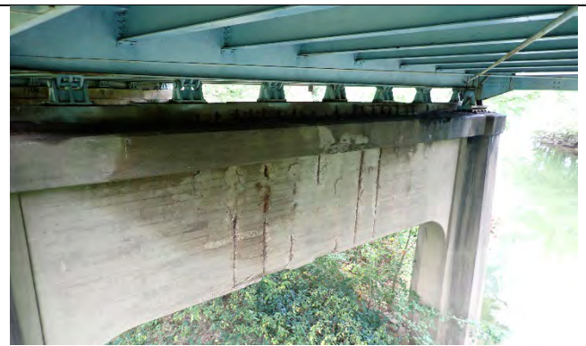
Photograph 55: Overall view of the rear face of Pier 2. Note extensive spalls and exposed reinforcing steel.
