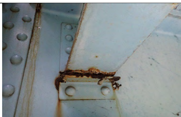
Photograph 26: Typical example of pack rust up to 1" thick between stringer bottom flanges and seat angles with up to 1/16" deep pitting to the stringer bottom flange underside.
