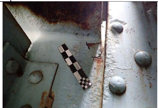
Photograph 36: Close up of Floor Beam 0 left truss cracks.
