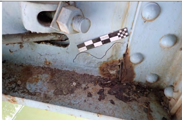
Photograph 42: Typical example of floor beam web pitting near the truss connection.
