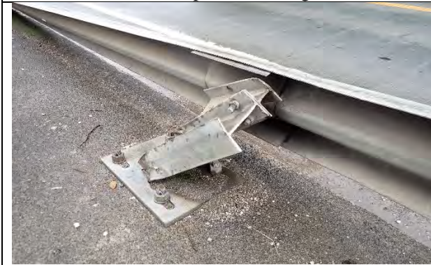
Photograph 21: Impact damage to first post for the right rear rail, Span 1, looking northwest.
