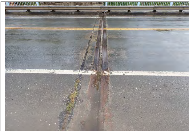
Photograph 11: Overall view of the Pier 3 joint. Note misalignment, debris in the joint, and armor damage. Looking south.
