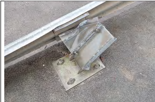
Photograph 19: Impact damage to the first post for the left forward rail, Span 4, looking southwest.
