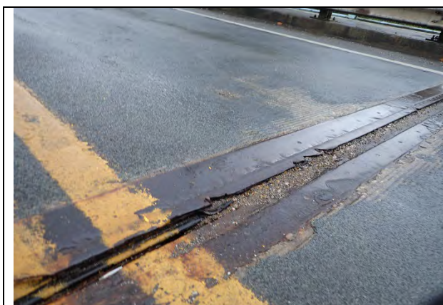
Photograph 9: Close up view of Far Abutment joint. Note typical slow plow damage and debris in the joint. Looking south.
