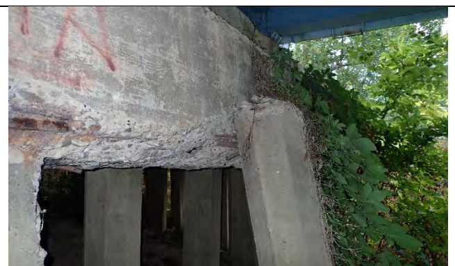
Photograph 53: Pier 3, the rear face pile under Beam 7 does not provide support for the cap. Looking southeast.
