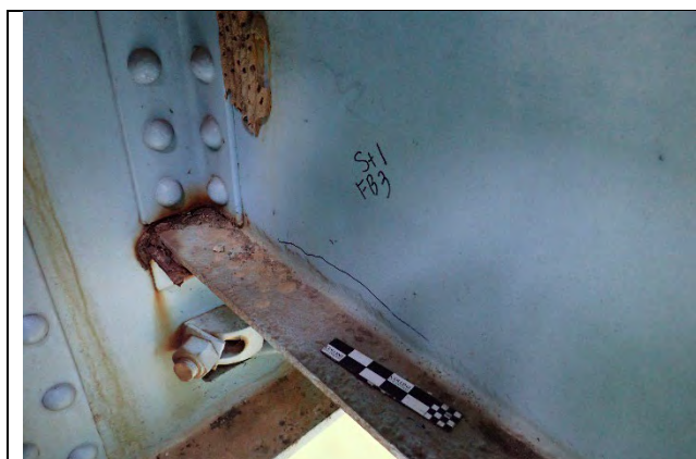
Photograph 25: View of the typical painted over pitting on the top of the bottom flange at the exterior face of the exterior stringer near floor beam connections. Floor Beam 3 Stringer 1 shown.
