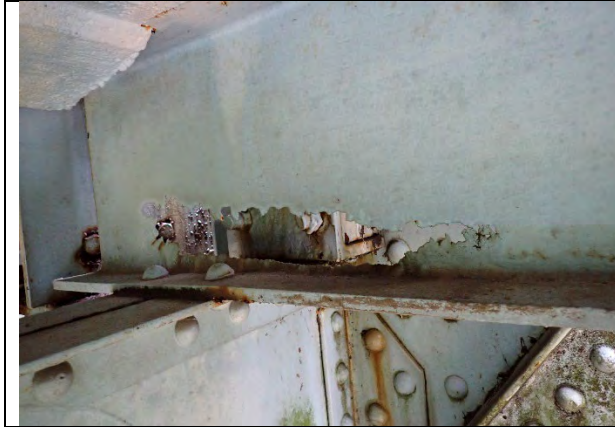
Photograph 27: General example of corrosion hole on the bottom of the sidewalk stringer web, Span 2.
