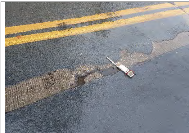
Photograph 3: General example of the deck top condition. Note worn away overlay and a small isolated spall on the top. No change this inspection.
