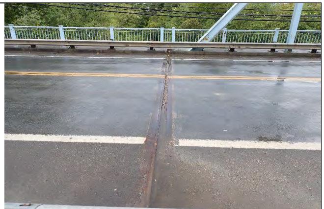
Photograph 12: Overall view of the Pier 2 joint. Note misalignment, debris in the joint, and armor damage. Looking south.
