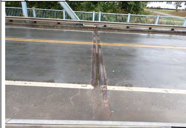
Photograph 13: Overall view of Pier 1 joint, looking south. Note debris in the joint.
