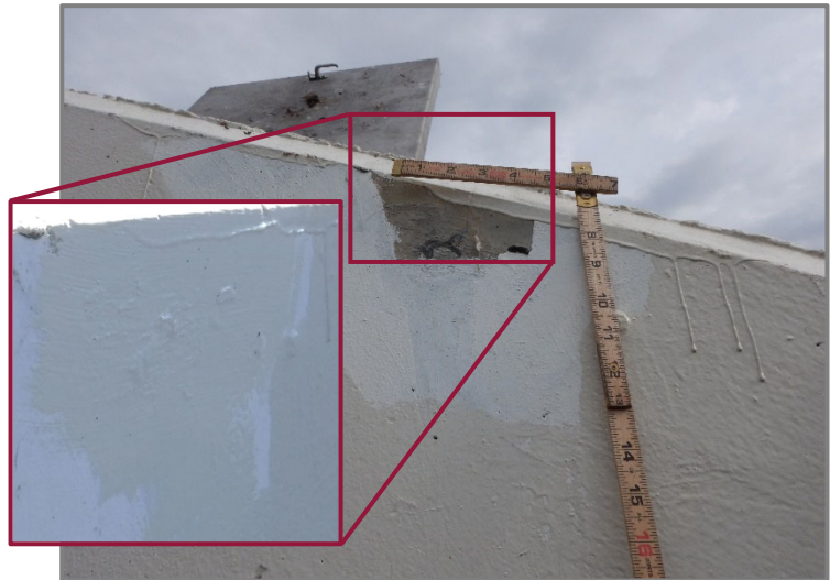
Photo 9 – Tower 4 south face at the top with an area that had a different color (looking north) and after areas were sealed (inset).
