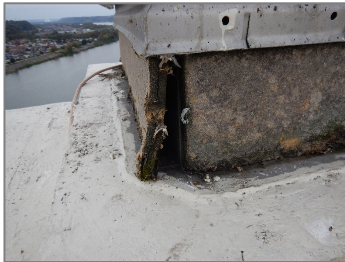
Photo 11 – Decayed boards around the exterior of the Tower 4 roof access hatch (looking east).
