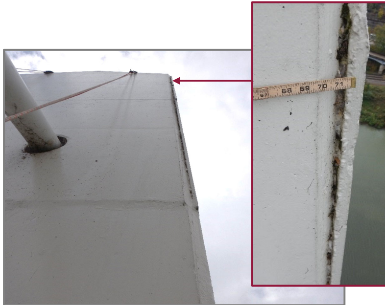
Photo 4 – Uneven forming of the west face of Tower 3 at the top, but no loose concrete was found (looking south at the northwest corner).
