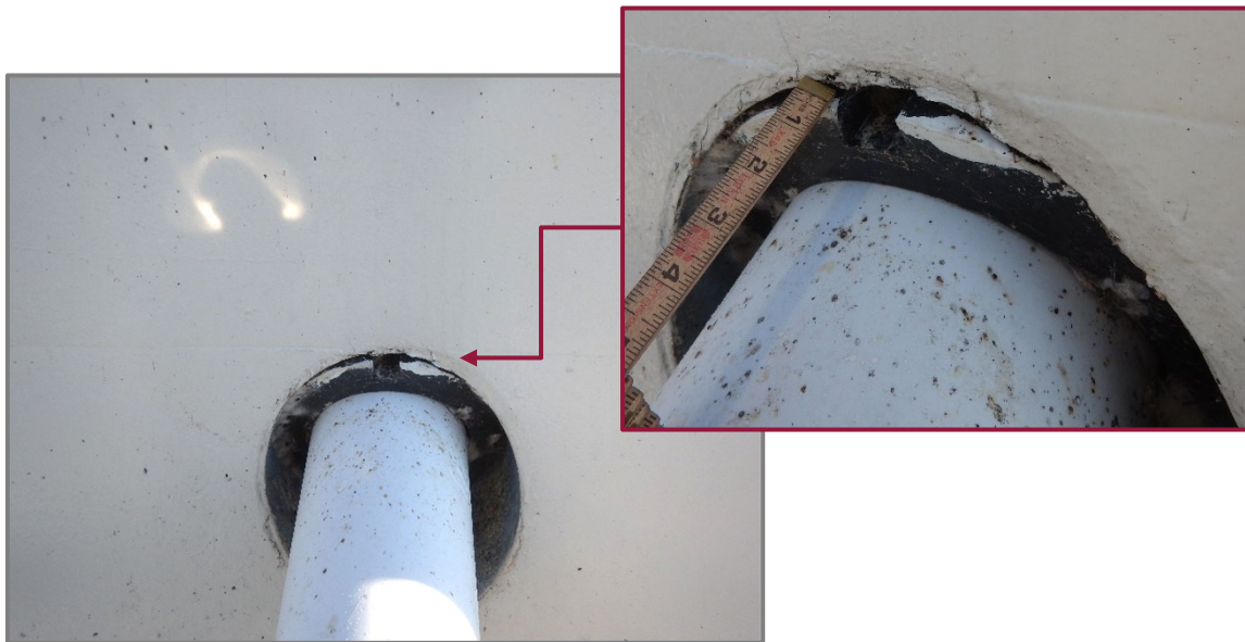
Photo 5 – Rubber gasket slightly extruded from steel guide tube (looking north at Cable B13E on the south face of Tower 3).
