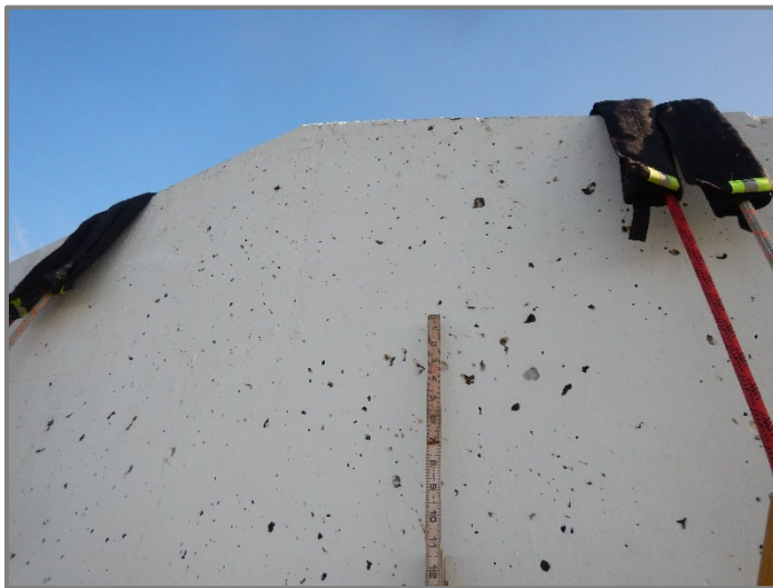
Photo 3 - Typical voids in the exterior faces of the towers (looking north at the south face of Tower 3 at the top).
