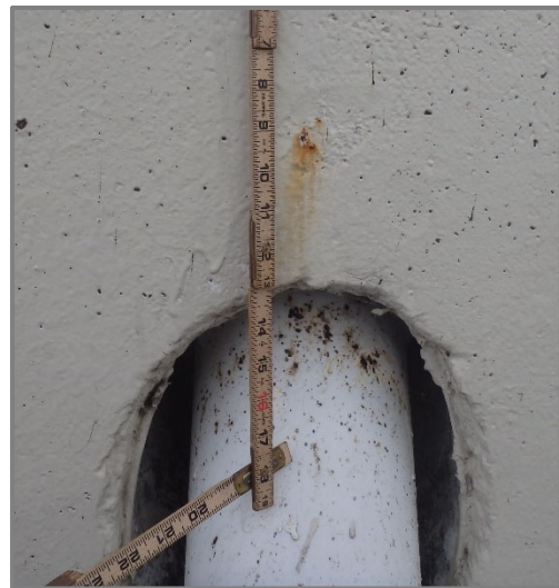
Photo 2 – Typical isolated area of minor rust staining (looking north at the south face of Tower 3 above Cable M19W).
