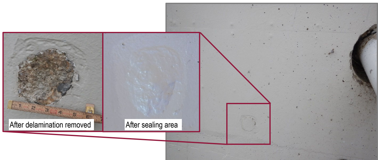
Photo 10 – Tower 4 south face in Segment 17 near Cable M30E with a delamination that was removed and sealed (looking north).
