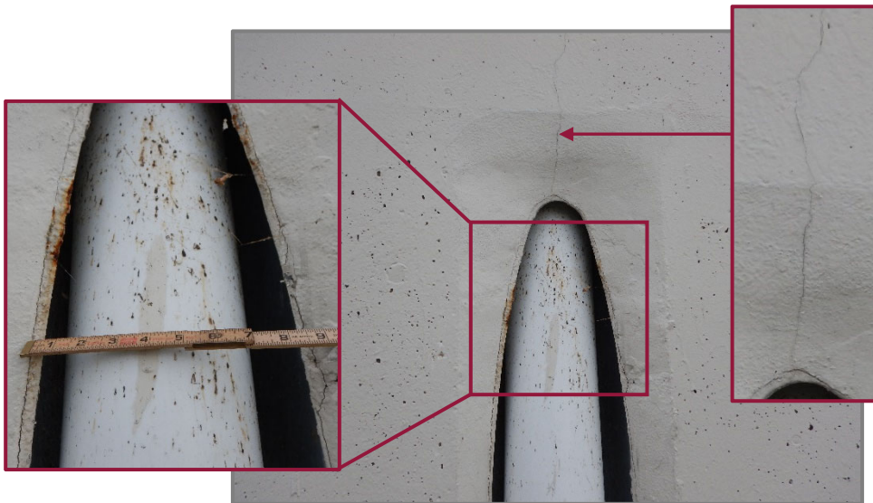
Photo 1 - Typical hairline crack above the anchor and cracking with rust staining around the guide tube (looking north at the south face of Tower 3 at Cable M16E in Segment 12).
