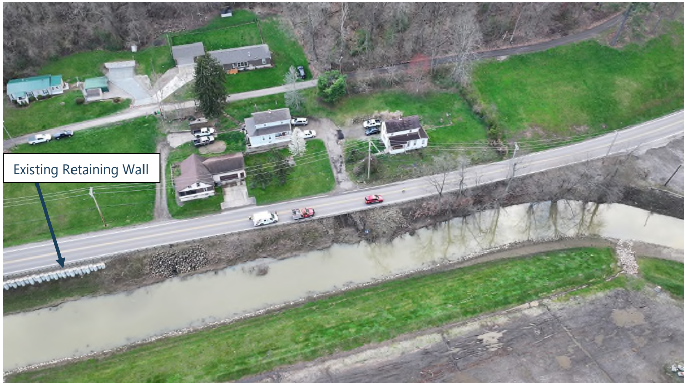
Figure 3-1 – Landslide Location and Adjacent Retaining Wall
