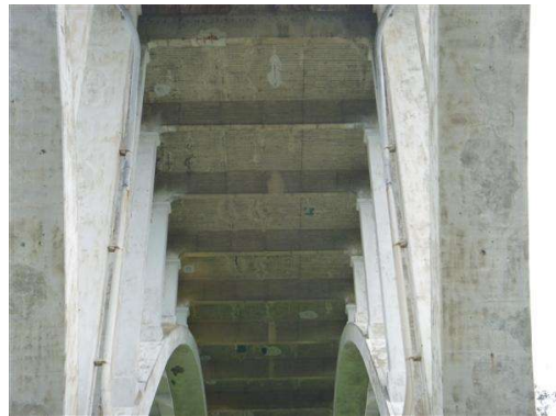
Photo 10 Typical condition of floorbeams
