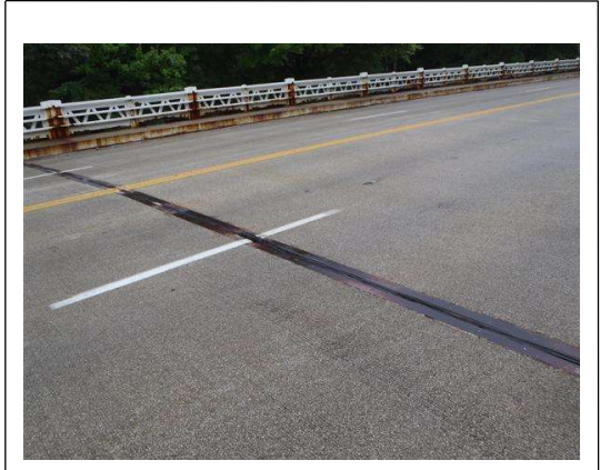
Photo 2 | Damaged seal 2
