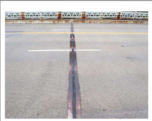
Photo 3 | Damaged seal
