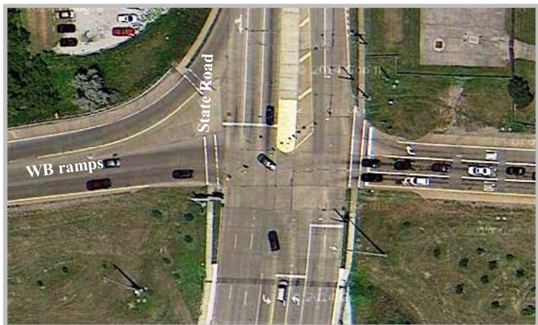
PHOTO 7: SR 94 AND I-480 WB RAMP INTERSECTION
