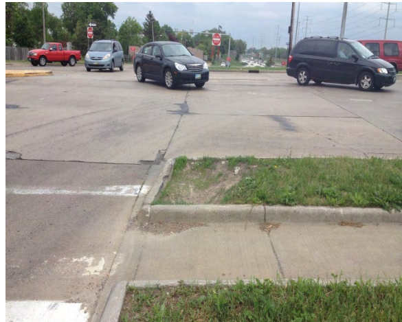
PHOTO 7: DAMAGED CURB IN SW QUADRANT
