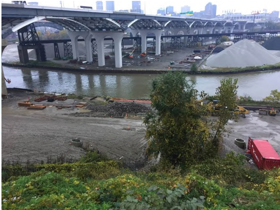
Figure 5. Aggregate stockpile near ODOT's east right-of-way fence (October 29, 2016).
