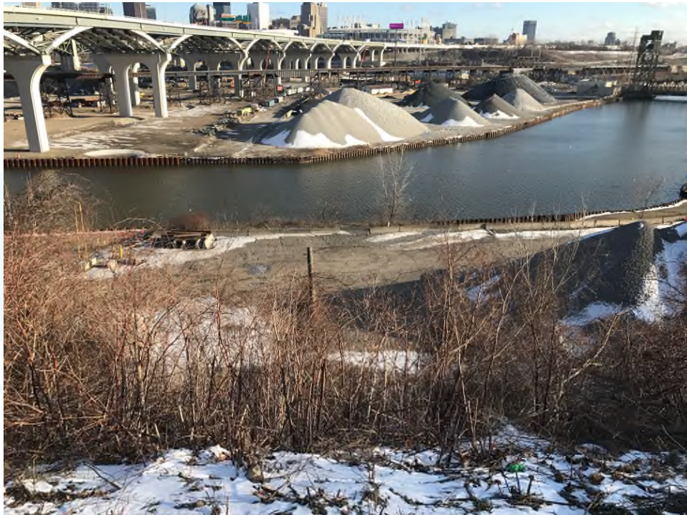
Figure 5. Aggregate stockpile near ODOT's east right-of-way fence (January 12, 2017).
