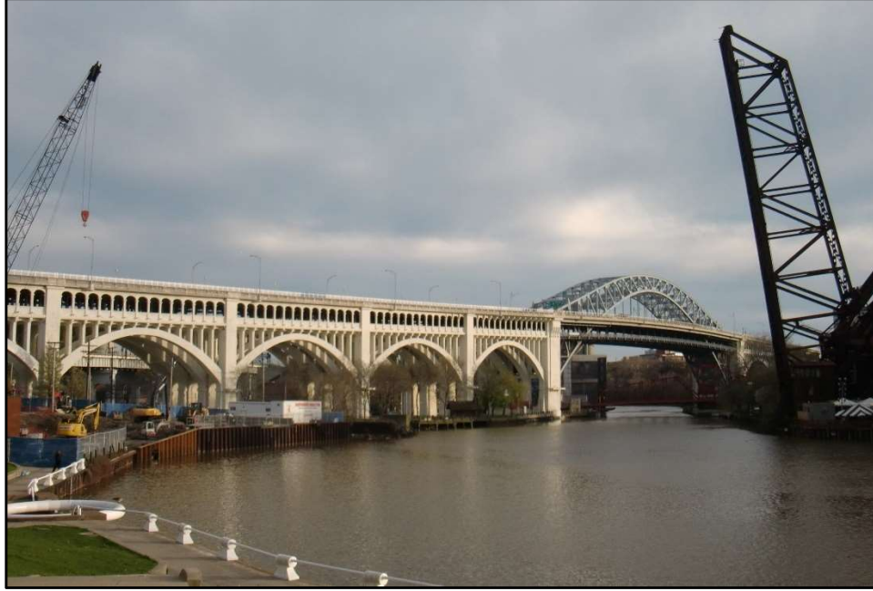
Photo 1 – North Elevation, Spans 4 through 8.
