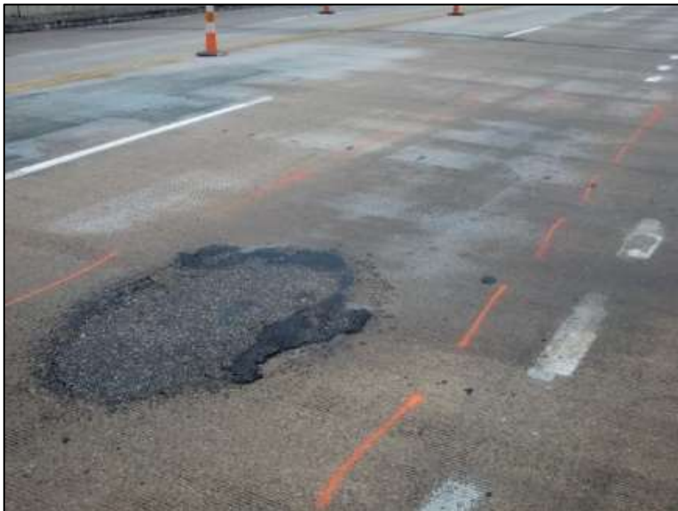
Photo 8 – Recent Wearing Surface Patching, Span 9.
