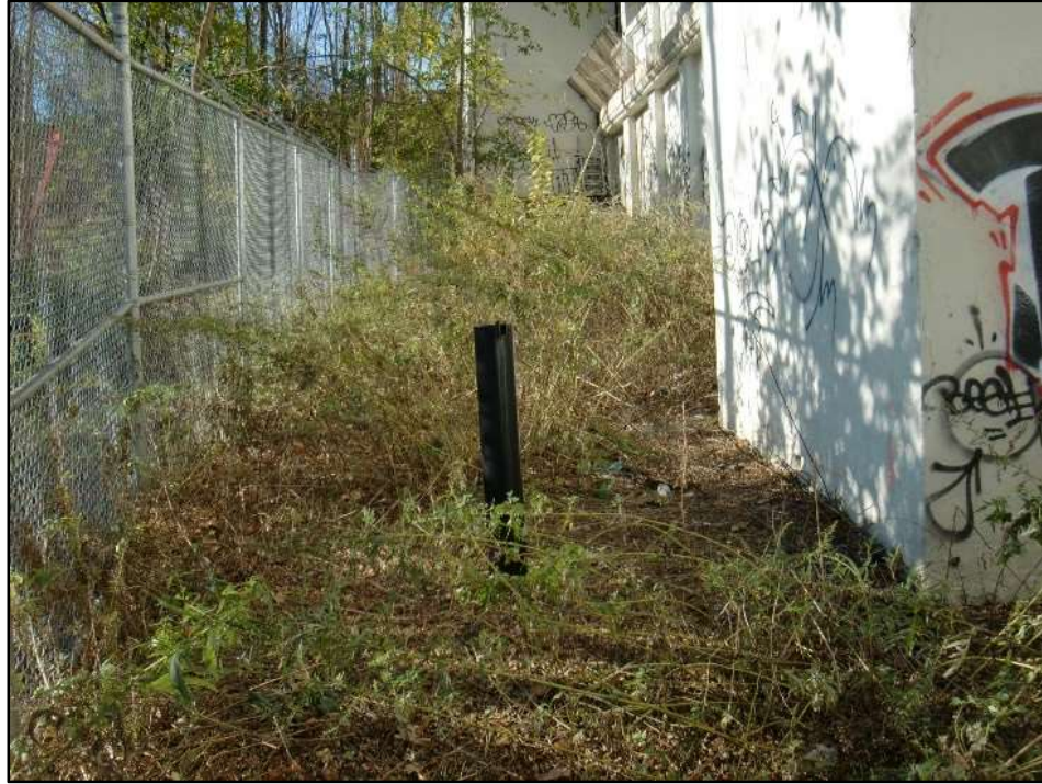
Photo 3– Slope Inclinometer, Tower B South.
