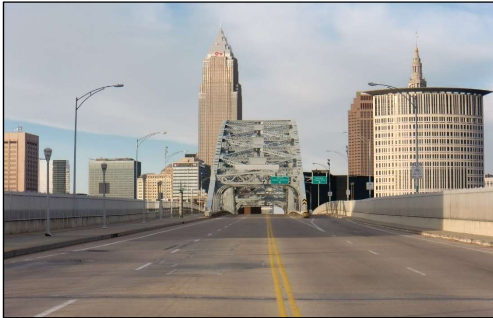
Photo 2 – Deck View, West Approach Spans, Looking East.
