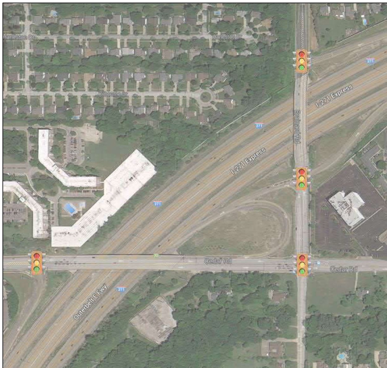
Figure 2. Aerial View of the Cedar Road/Brainard Road/I-271 Interchange.
