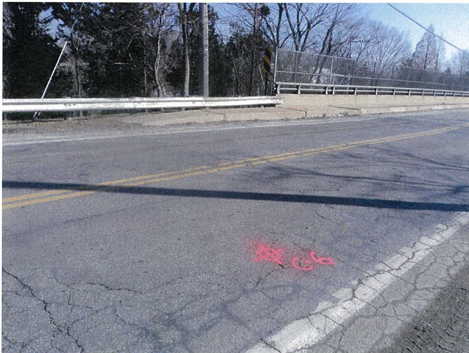
Pavement Photo C-6
