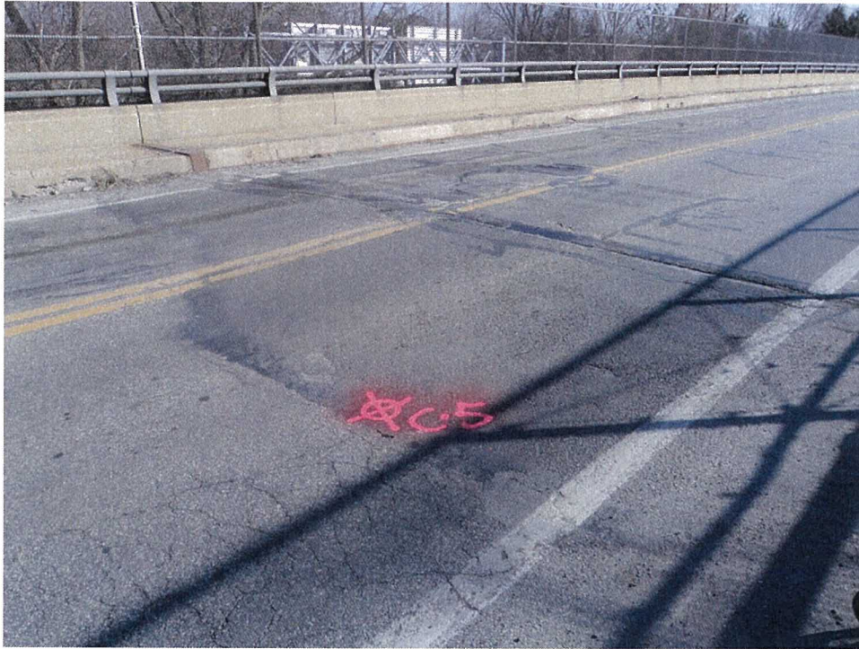
Pavement Photo C-5
