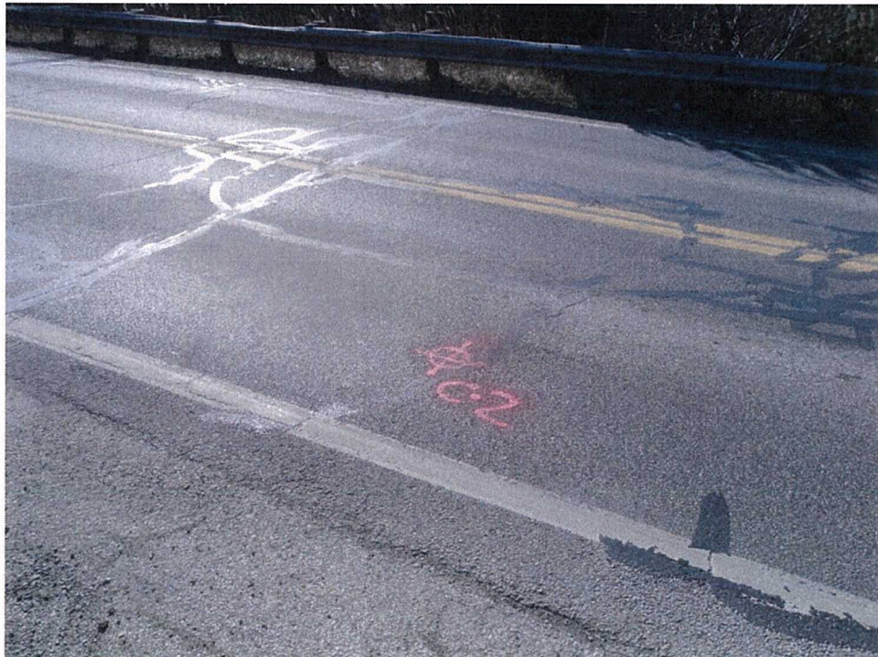
Pavement Photo # C-2
