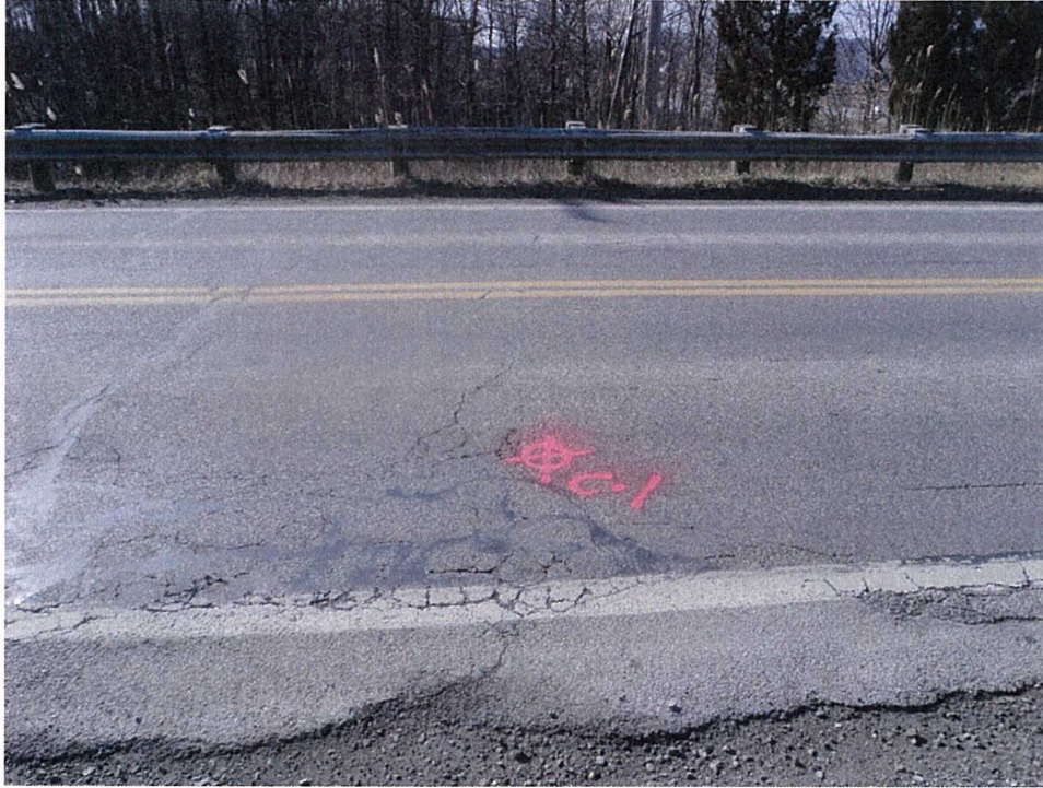
Pavement Photo # C-1
