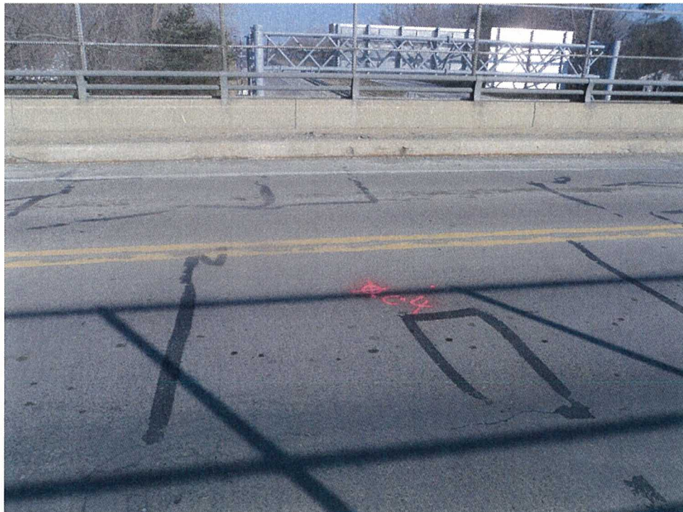
Pavement Photo C-4
