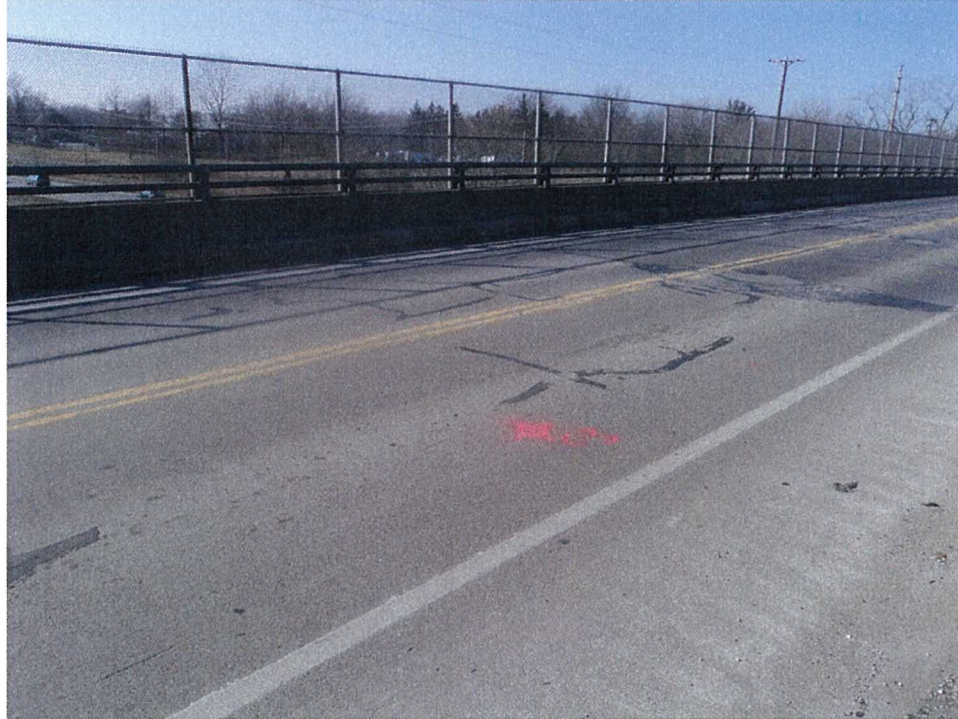
Pavement Photo C-3
