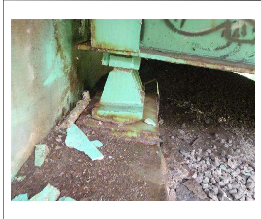
Photo 2 Evidence of edge spalls occurring in the tops of the backwalls.
