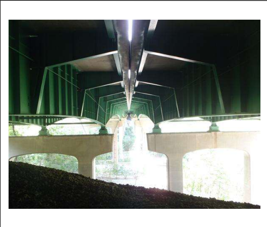
Photo 1 Typical good paint and steel condition.
