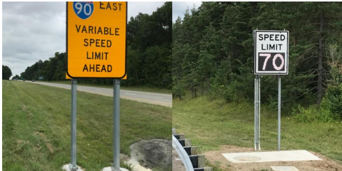
Figure C-5. Variable Speed Limit Signs on I-90
