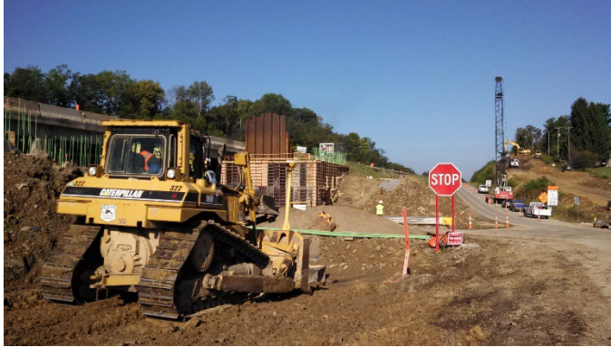
Grading near an active intersection, with phased bridge construction underway in the background
