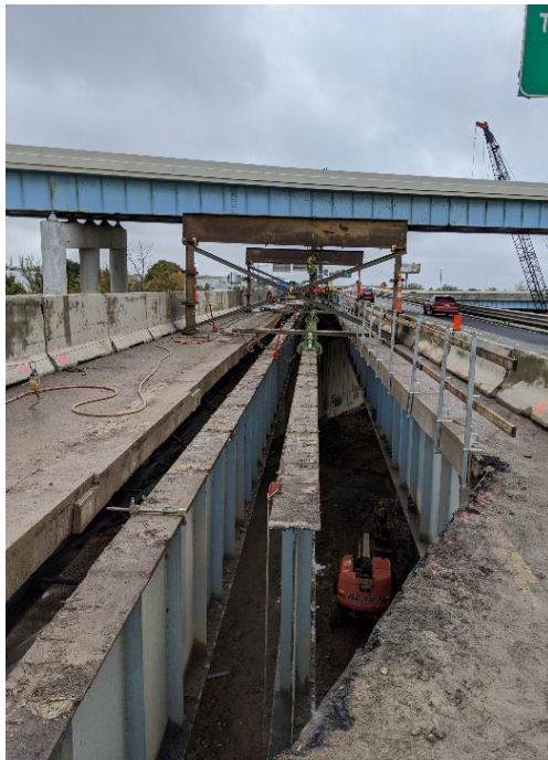
Custom chain-hoist system being used to remove a bridge girder in tight ROW conditions.
