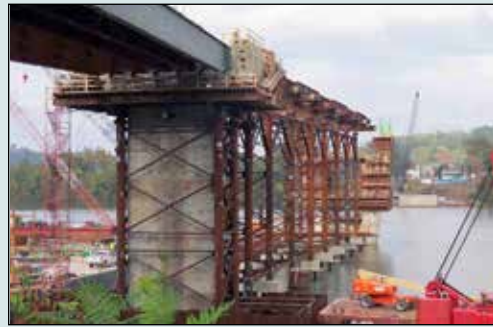
Brayman's custom designed modular falsework system at Ironton-Russell.
