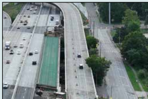
Part-width construction of mainline bridge.
