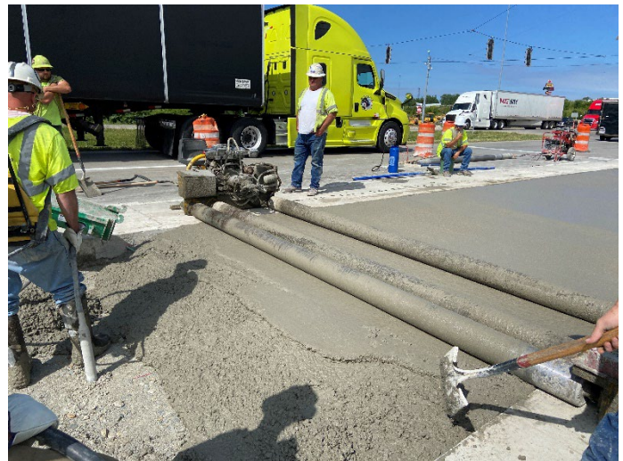
Three-tube roller screed – Note the paste production at the top of the slab
