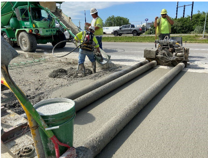
Three-tube roller screed – Note the paste production at the top of the slab
