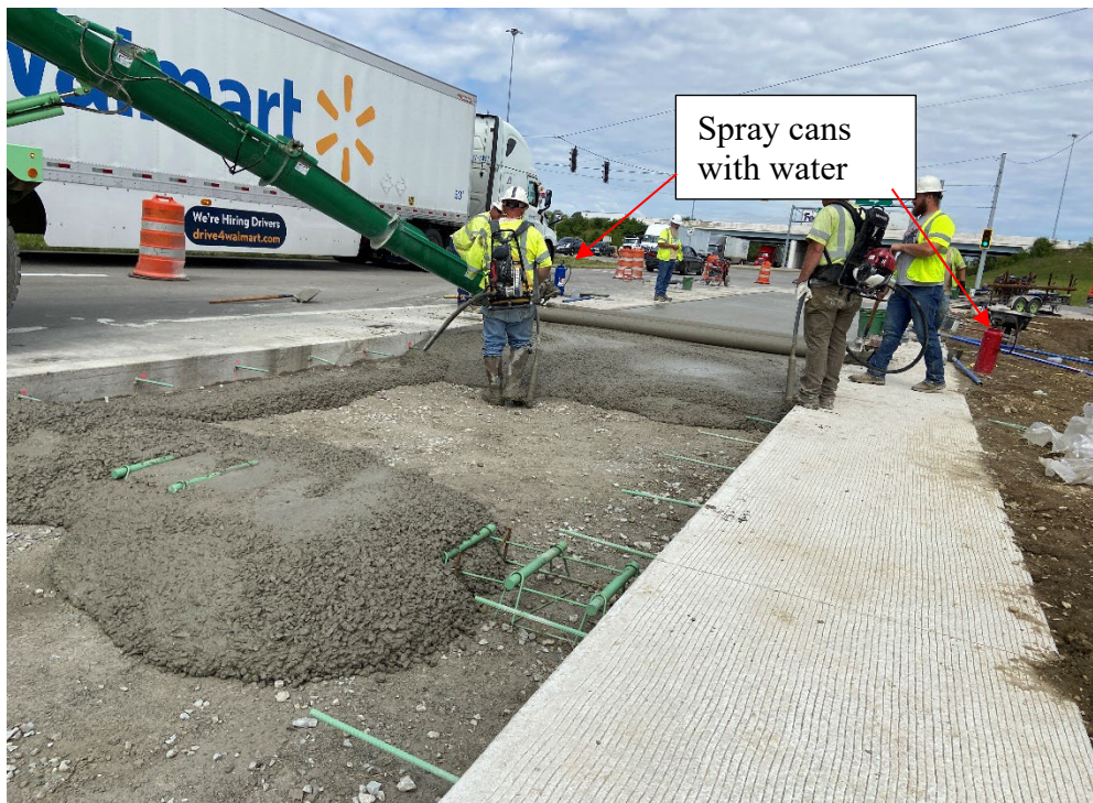
General view of the paving operation. Note the blue and red spray cans. These contained water.
