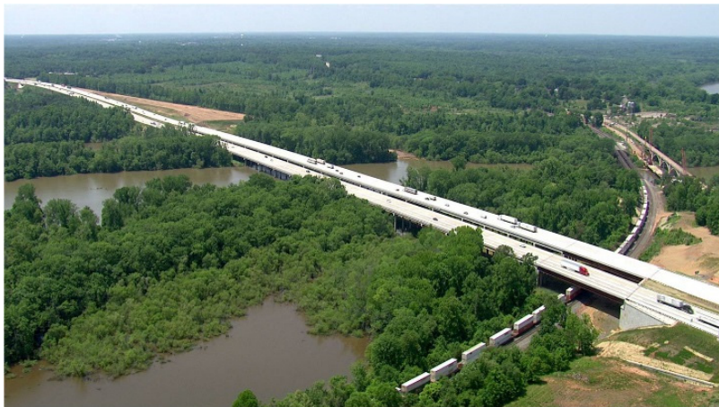
STV’s I-85/Yadkin River Bridge (high speed RR crossing, total of 5 tracks including future rail)
