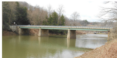
PA Rapid Bridge Replacement Program P3 Various Locations, PA | $899M
