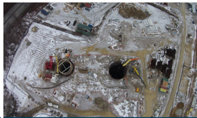
Easterly Tunnel Pump Station Cleveland, OH | $73M
