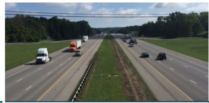
I-71, 6-Lane Upgrade DB - Project #1 Morrow County, OH | $54M
