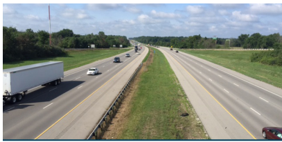
I-71 Golden Spike DB - Project #3 Morrow County, OH | $53M
