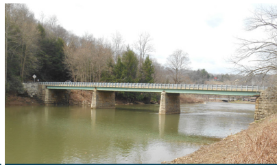
PA Rapid Bridge Replacement Program P3 Various Locations, PA | $899M
