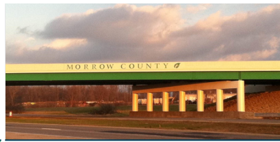
I-71, 6-Lane Upgrade DB - Project #2 Morrow County, OH | $50M
