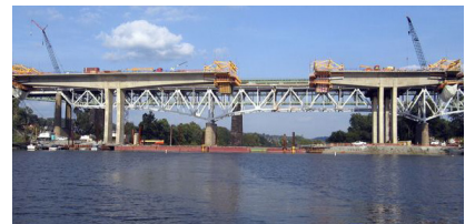
Allegheny River Bridge Cheswick, PA | $190M
