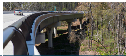
Intercounty Connector, Contract A DB Montgomery County, MD | $484M
