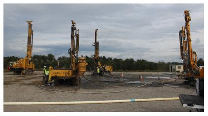
was especially concerning to Chevron due to the strict tolerances of settlement for the drilling equipment. Chevron contacted HCP for a solution to install the proposed drill rig operation on the existing subgrade material. HCP developed an innovative permeation/compaction grouting program to fill the subsurface voids.
