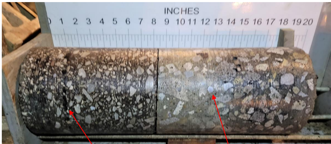
Layer with higher bitumen content
