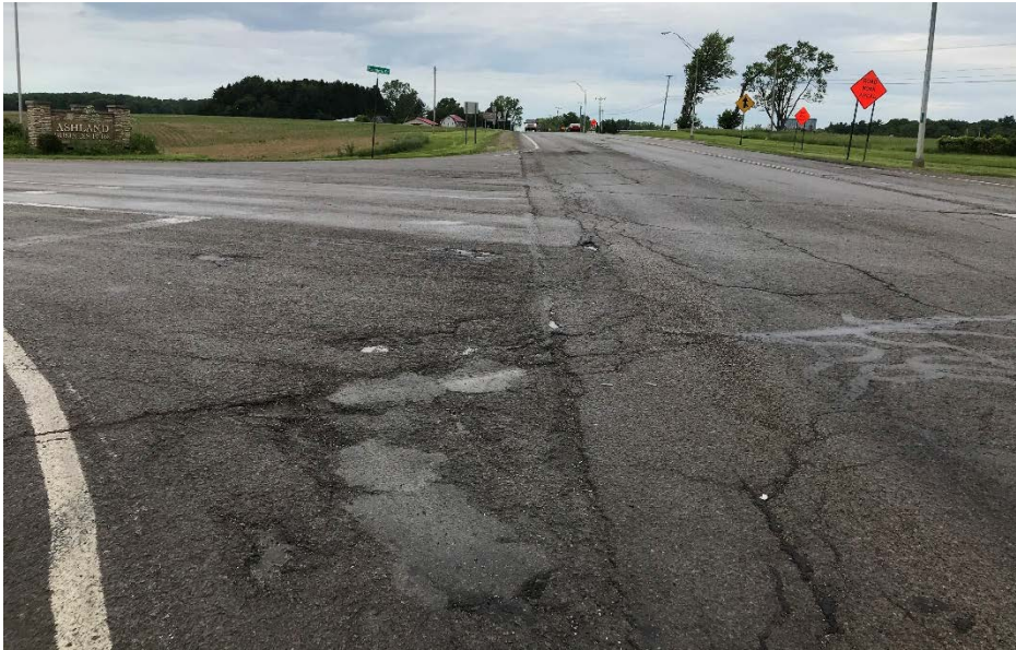
Photograph 2: US 250 / SR 60 / Faultless Drive Intersection (facing North)
