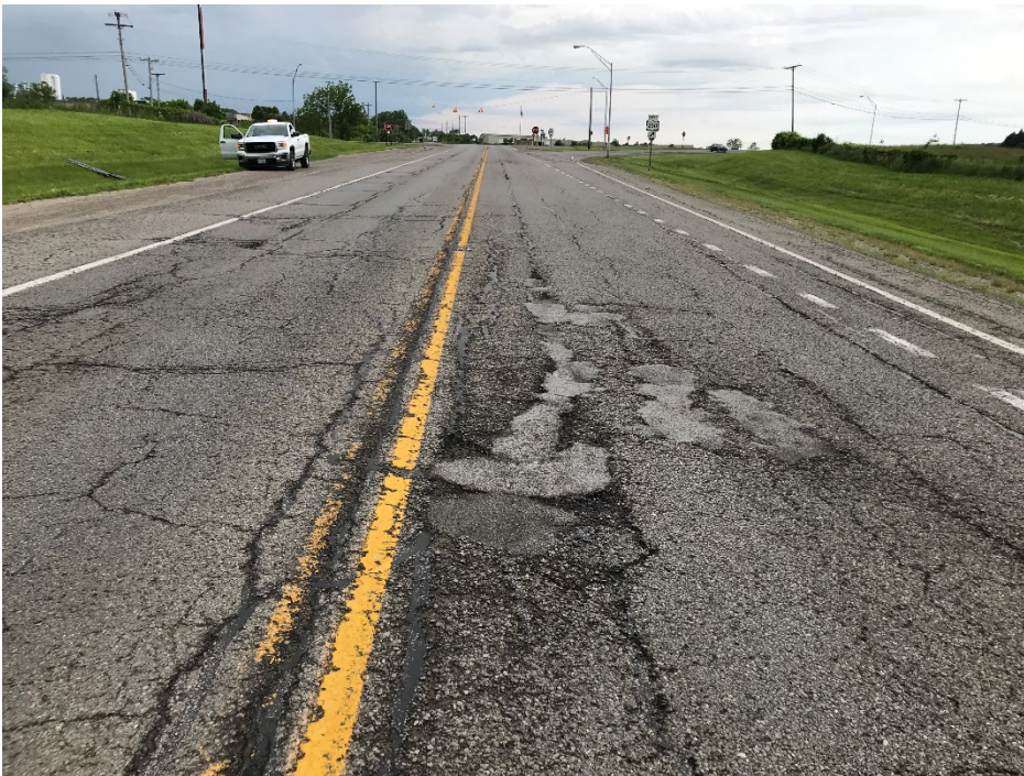
Photograph 3: East of US 250 / SR 60 / Faultless Drive Intersection (facing West)
