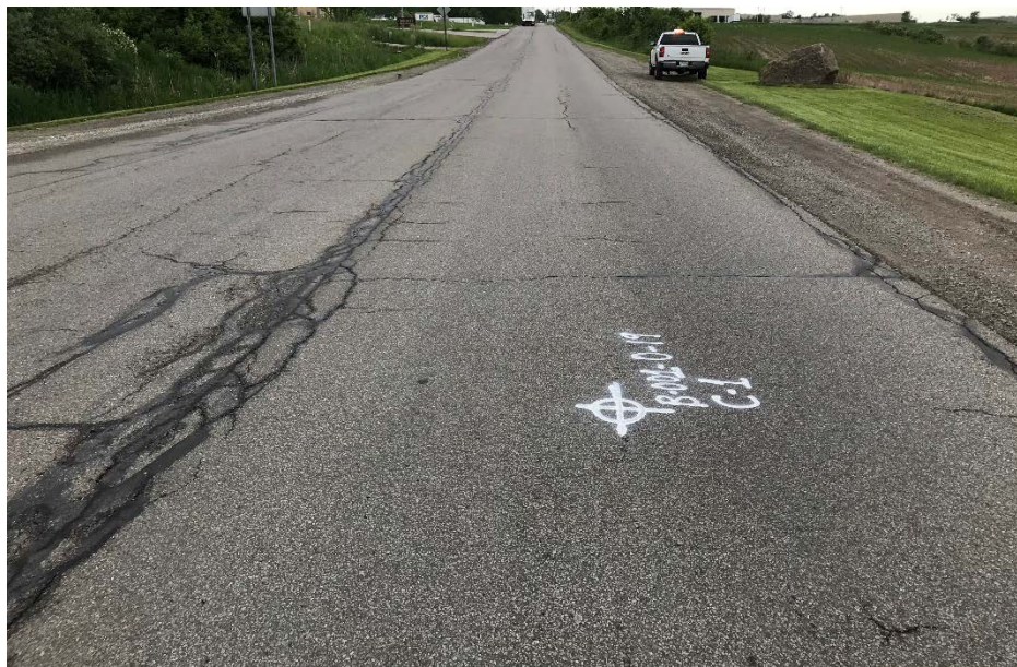
Photograph 1: Faultless Drive (West of US 250 / SR 60 / Faultless Drive Intersection)
