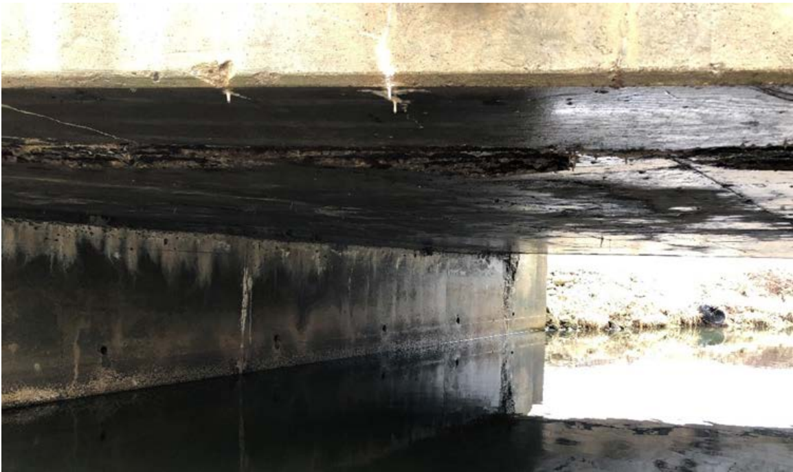
Photograph 1: Reinforced Concrete Bridge Deck and Full Height Abutments
