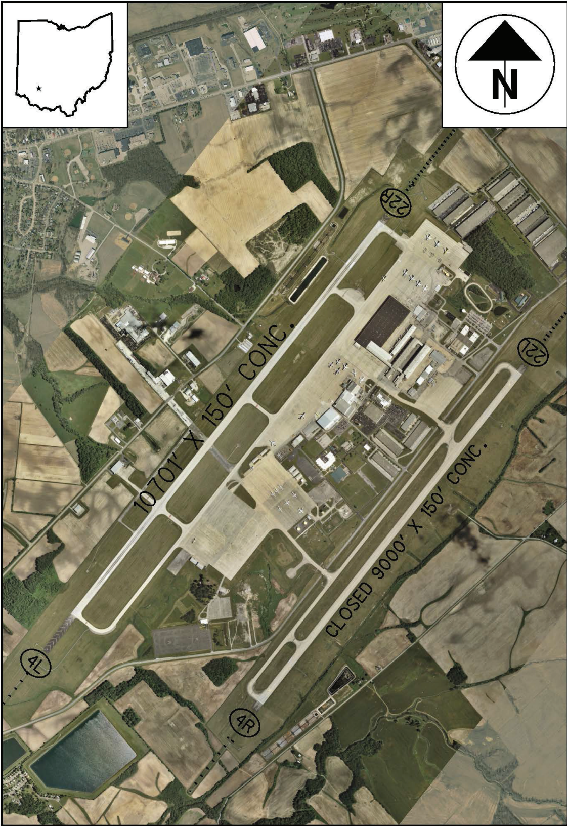
Imagery Source: ODOT Imagery Date: 06/08/16
