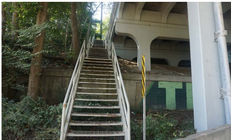
Photograph 5: Retaining wall and slope along proposed wall alignment
