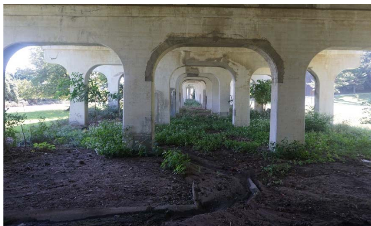
Photograph 1: Drainage area under existing bridge near Bent No. 1
