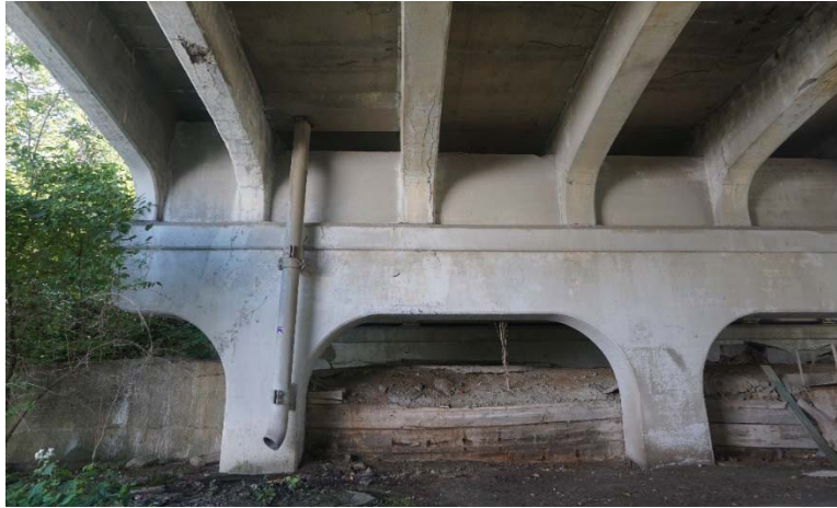
Photograph 4: Walls near existing Bent No. 48 and 49
