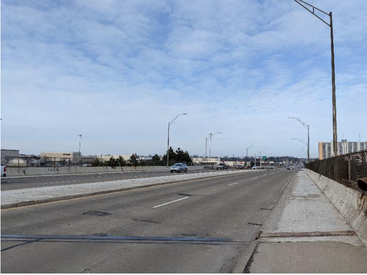
PHOTO 1 Looking north at CUY-252-4.370 bridge
