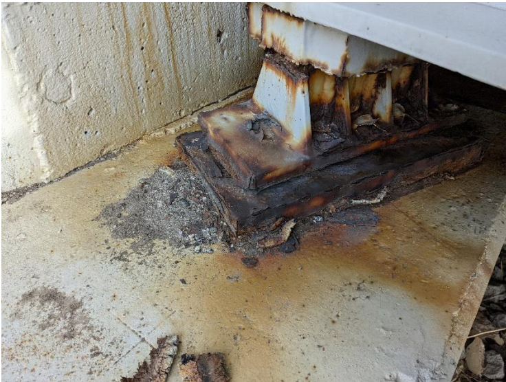
PHOTO 2 Looking down at rocker and beam seat, all metal.
