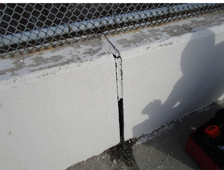
PHOTO 9 Parapet railing on the deck. Sample taken of expansion joint.
