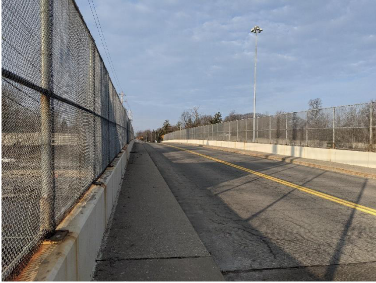
PHOTO 1 Looking west at CUY-271- 15.410 bridge
