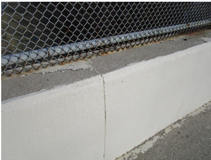
PHOTO 8 Parapet railing on the deck. Sample taken of joint compound.
