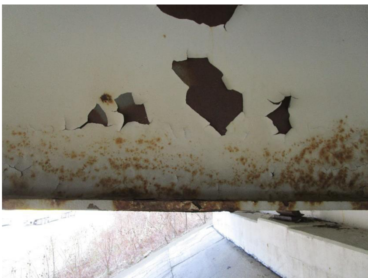
PHOTO 3 Underside of bridge. Paint samples collected.
