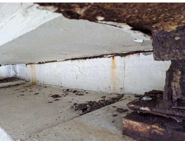
PHOTO 6 Expansion joint on east back wall. Sample taken here.
