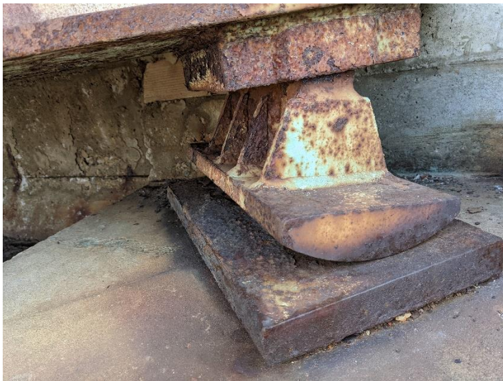
PHOTO 5 Rocker and bearing plate, (all metal)
