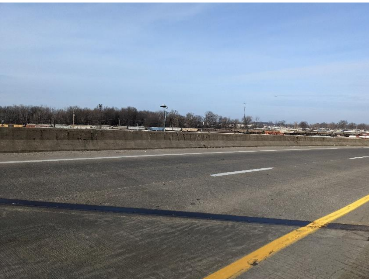
PHOTO 6 Topside of structure facing northwest.
