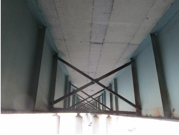
PHOTO 1 Looking north at CUY-480-0.000 bridge. No utilities affixed to the structure.
