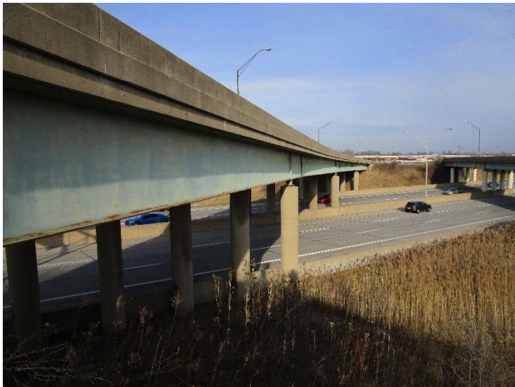
PHOTO 3 Facing north looking at the east side of the structure.
