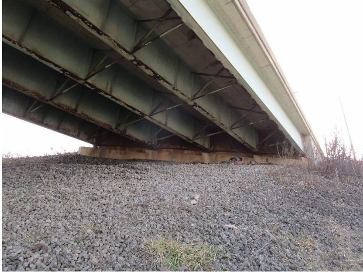
PHOTO 4 Underside of structure. South end.
