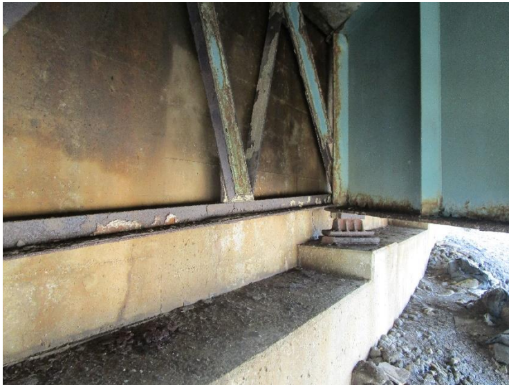
PHOTO 2 Looking at the south end wall. Concrete and steel only.
