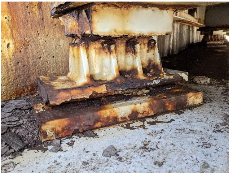
PHOTO 6 View looking at the rocker and bearing pad that is all metal.
