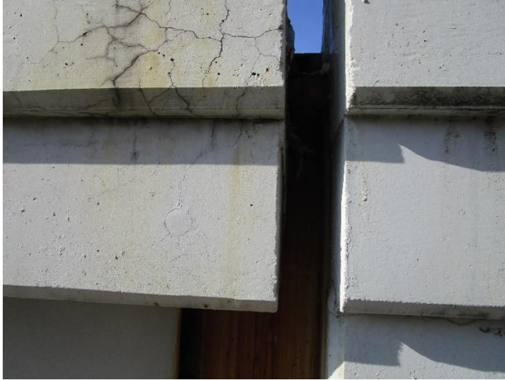
PHOTO 10 View looking at the northside of structure, where mastic sealant sample from 2" electrical conduit line was taken.
