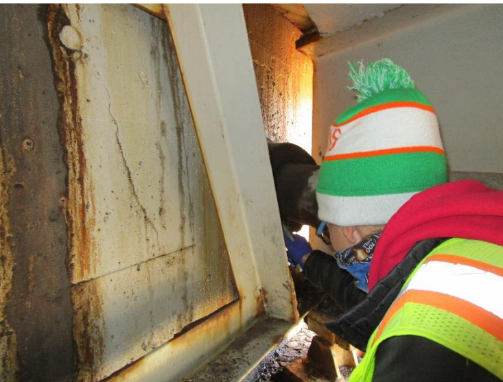
PHOTO 12 View looking at north back wall 6 5/8" gas line packing material.
