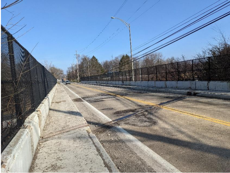
PHOTO 1 Looking north at CUY-480-4.440 bridge
