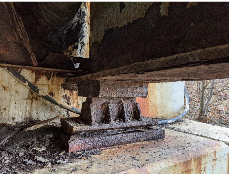
PHOTO 6 View looking at the bridge seat that is all metal.
