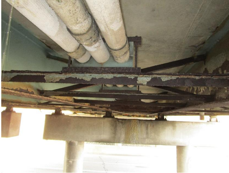
PHOTO 7 View looking at underside of structure. Transite pipe present.
