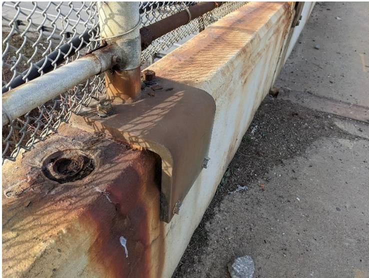
PHOTO 2 Vandal fence mounting bracket. Sample taken from caulking.
