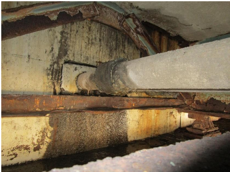
PHOTO 3 Transite pipe and coupler. Sample taken from coupler.
