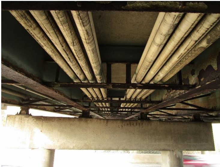
PHOTO 5 View looking at underside of structure. PVC pipes present.
