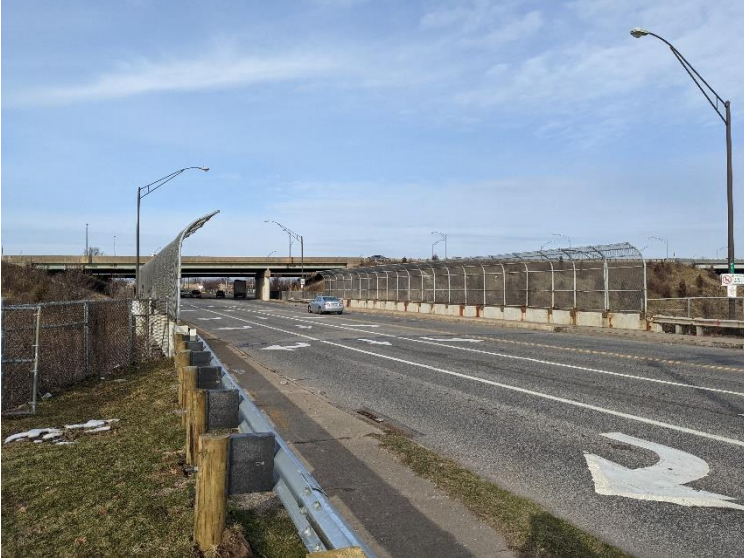
PHOTO 1 Looking north at CUY-480-7.920 bridge
