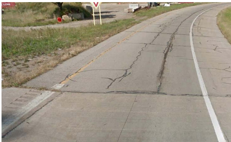
Photograph 11: Overall Pavement Condition of Ramp E-N
