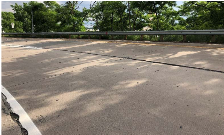
Photograph 6: Overall Pavement Condition of Ramp 7-7C
