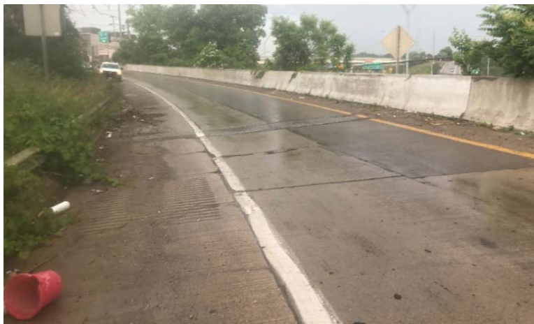
Photograph 8: Overall Pavement Condition of Ramp B-C
