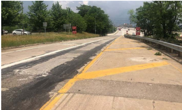
Photograph 7: Overall Pavement Condition of Ramp C-7
