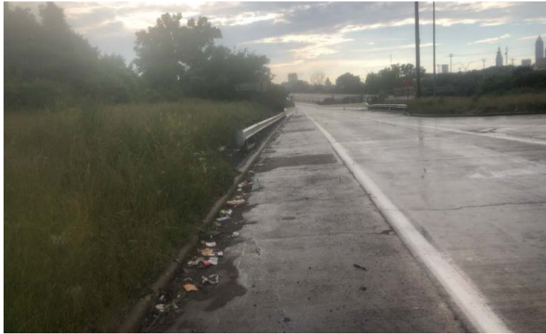
Photograph 9: Overall Pavement Condition of Ramp C-B
