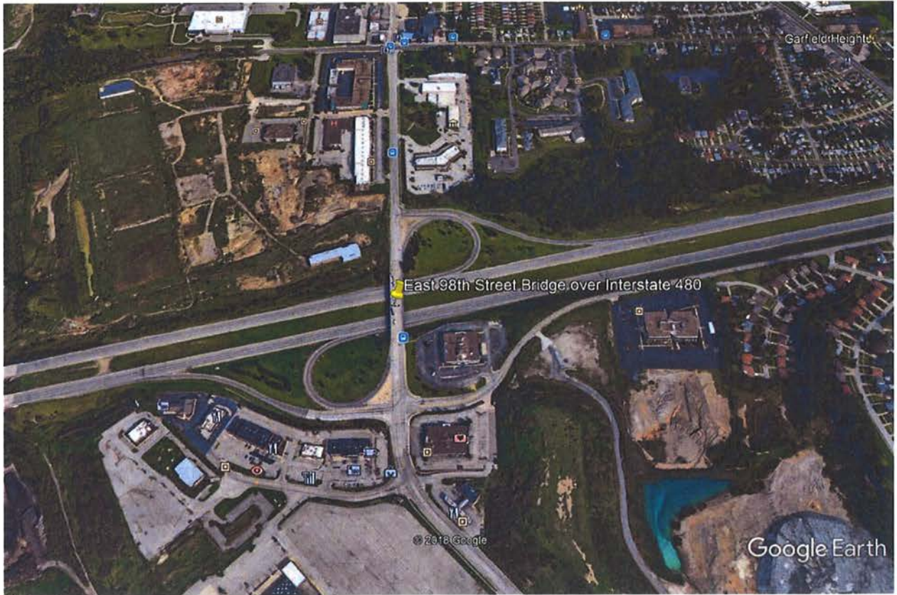
Aerial of the East 98 th Street Bridge over Interstate 480 Garfield Heights, Ohio
