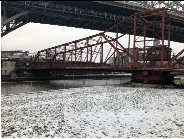
Photo 1: View of Center Street Swing Bridge
