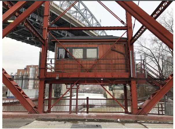
Photo 2: View of Operators House Facing West
