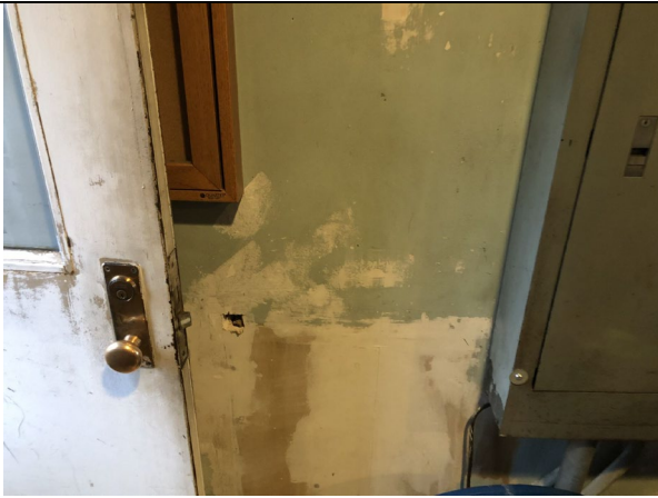
Photo 3: View of Drywall and Joint Compound Located in the in Operator's House
