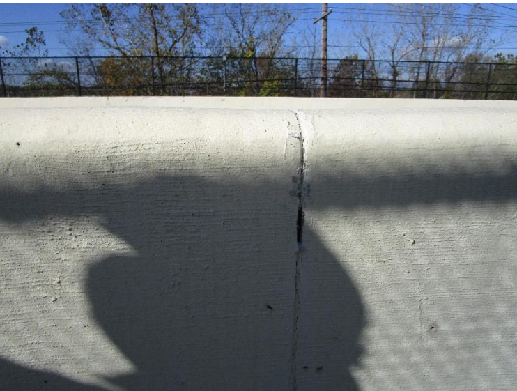
PHOTO 6 View looking at typical parapet joints.
