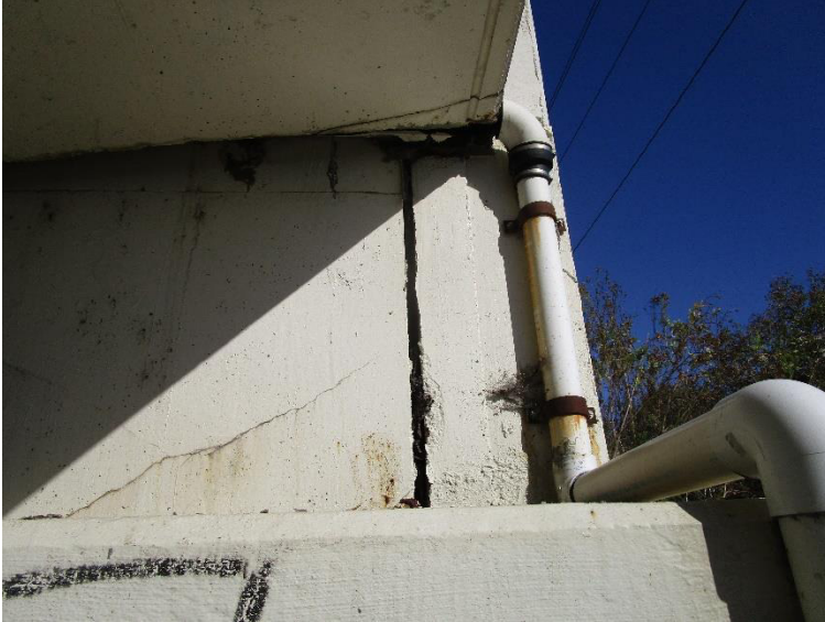
PHOTO 7 View looking at abutment, scupper drain, and expansion joint material
