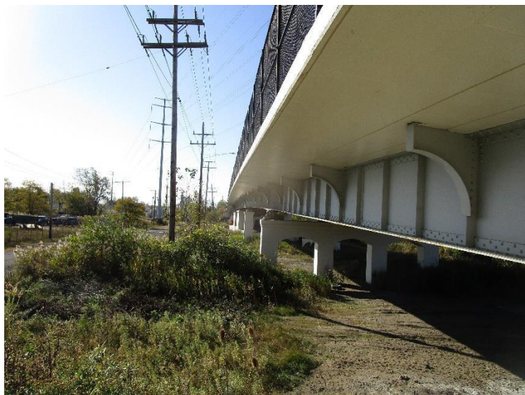
PHOTO 9 View of outer beam-line, sidewalk overhang and vandal fencing
