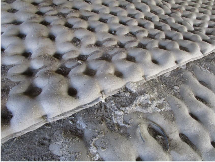
PHOTO 4 Grout filled slope protection matting.
