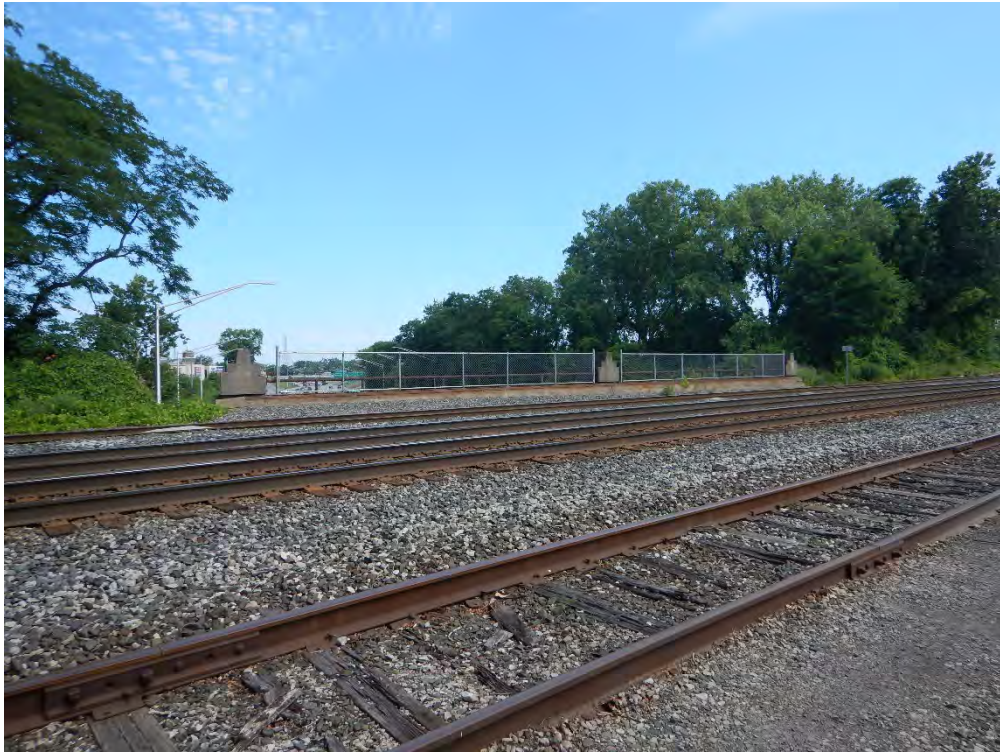
Photo 5: Existing CSX bridge over IR-77, facing north.
