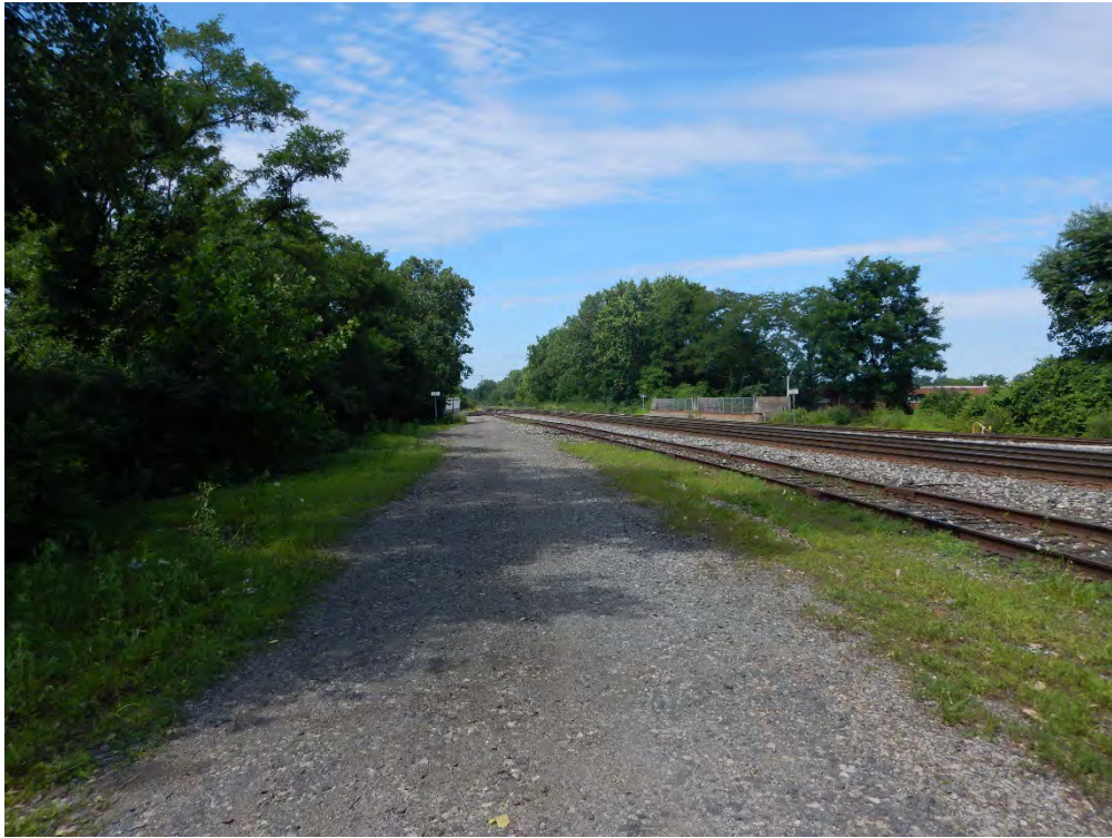
Photo 1: View of existing CSX bridge over IR-77, facing east.
