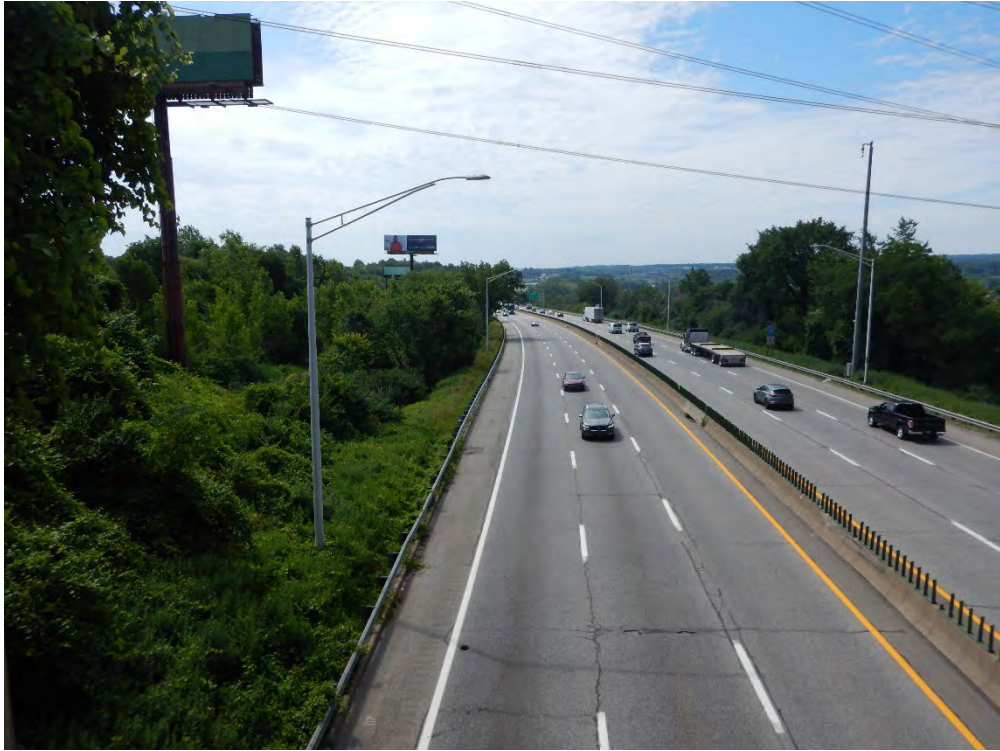
Photo 2: View of Interstate 77 from the CSX bridge, facing south.
