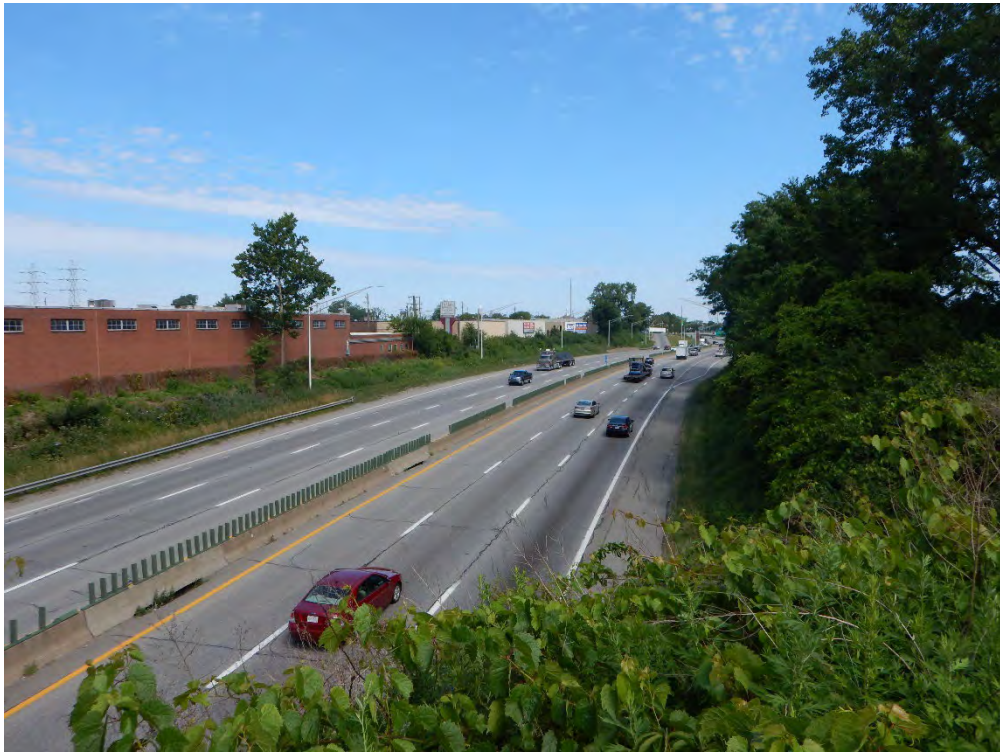
Photo 6: View of IR-77 from CSX bridge, facing north.
