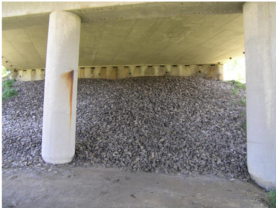
Photograph 3: FRA-71-0308 NB Pier 3 and Forward Spill Through
