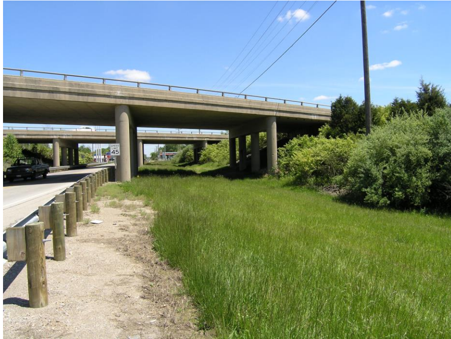
Photograph 2: FRA-71-0308 NB Piers 2 and 3.
