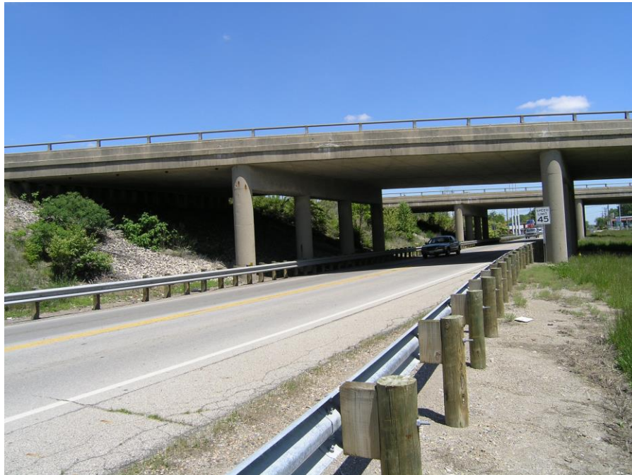
Photograph 1: FRA-71-0308 NB Piers 1 and 2.
