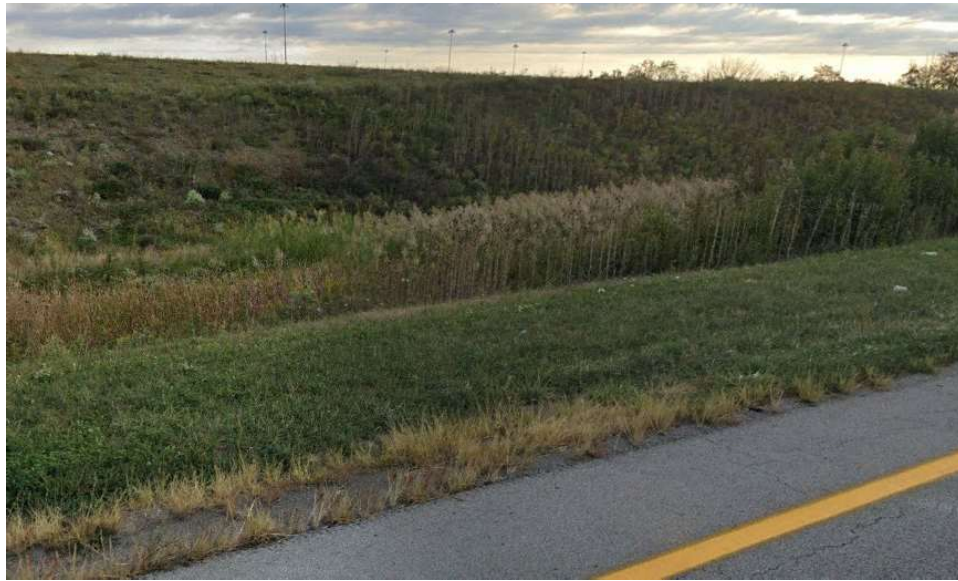
Photograph 2: Signs of Standing Water in Drainage Ditch
