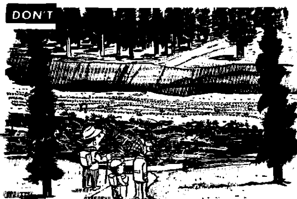
EPM No. 10. —Where game trails or hiking trails cross construction areas, such trails shall not be covered by debris and shall be maintained in a safe and passable condition at all times.
