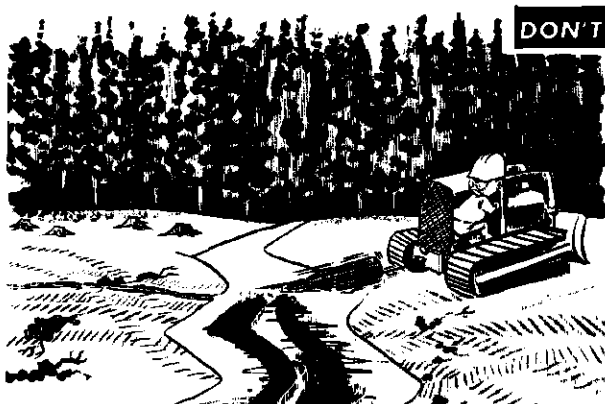
EPM No. 19. —The use of equipment within streams shall be held to that necessary for preparing a base for culverts and for channel diversion only.
