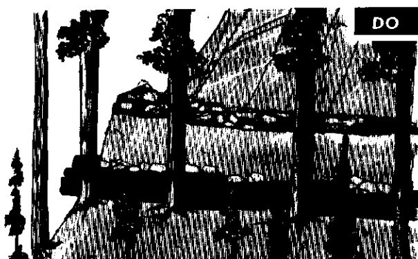
EPM No. 13. —The contractor shall erect log barriers in specified locations to prevent excavated material from escaping down the slope. The log barriers shall be placed at the edge of the cleared area or in other locations up the slope as approved by the Contracting Officer.
