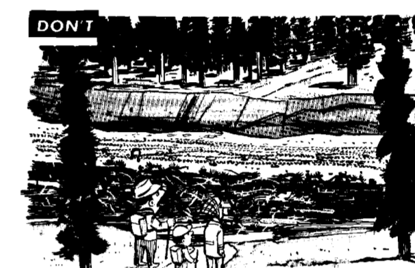
EPM No. 10. —Where game trails or hiking trails cross construction areas, such trails shall not be covered by debris and shall be maintained in a safe and passable condition at all times.
