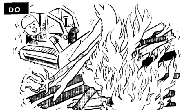
EPM No. 24. —Except as restricted by the Fire Control Officer, burning shall assure continuous, rapid and complete combustion. To meet this requirement, burning piles shall be kept under constant attendance by heavy equipment and operators who shall stack or push in burning piles from the edges, or shall feed fire with additional combustibles.
