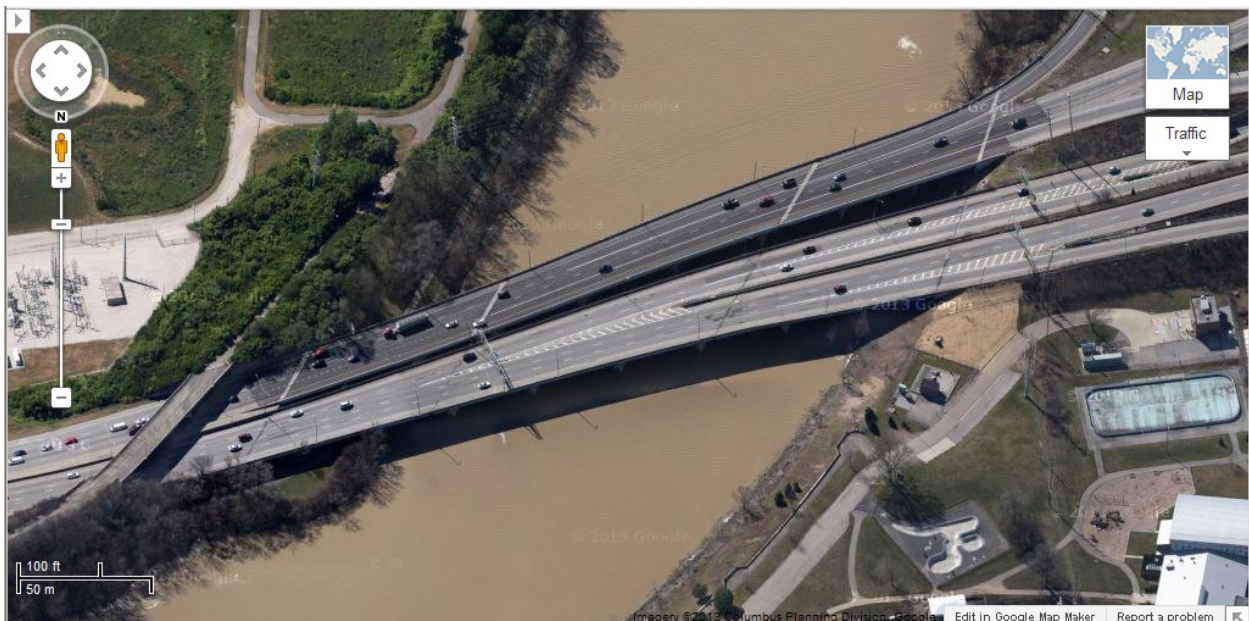
Figure 8: View: Existing Bridge: Upstream looking Downstream
