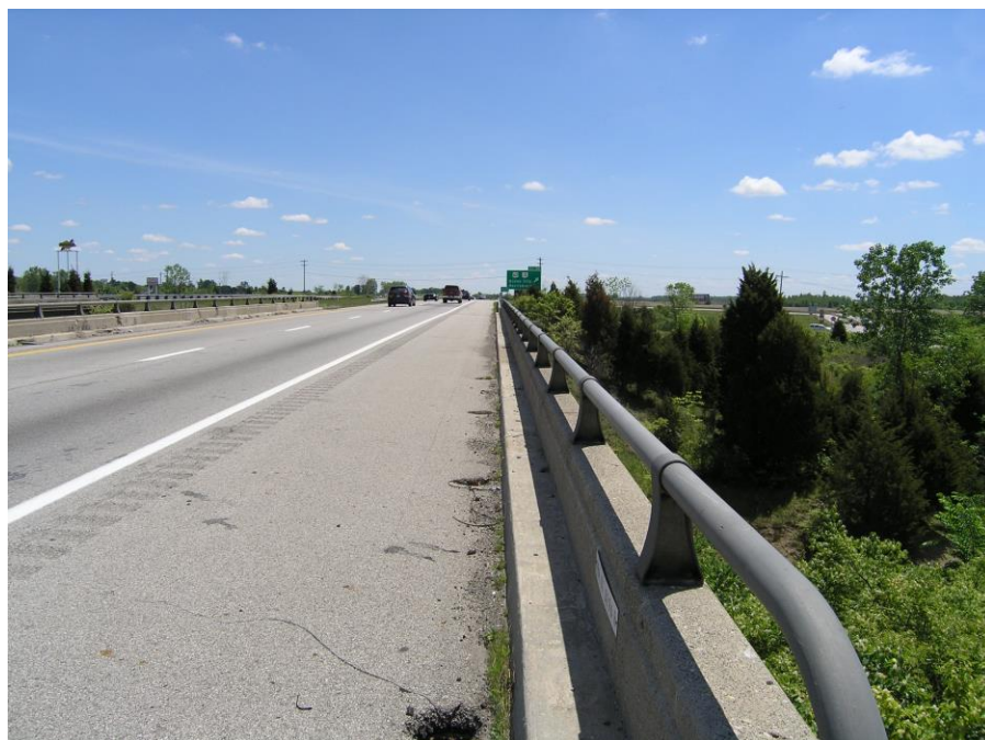
Photograph 1: NB FRA-71-0296 looking north.
