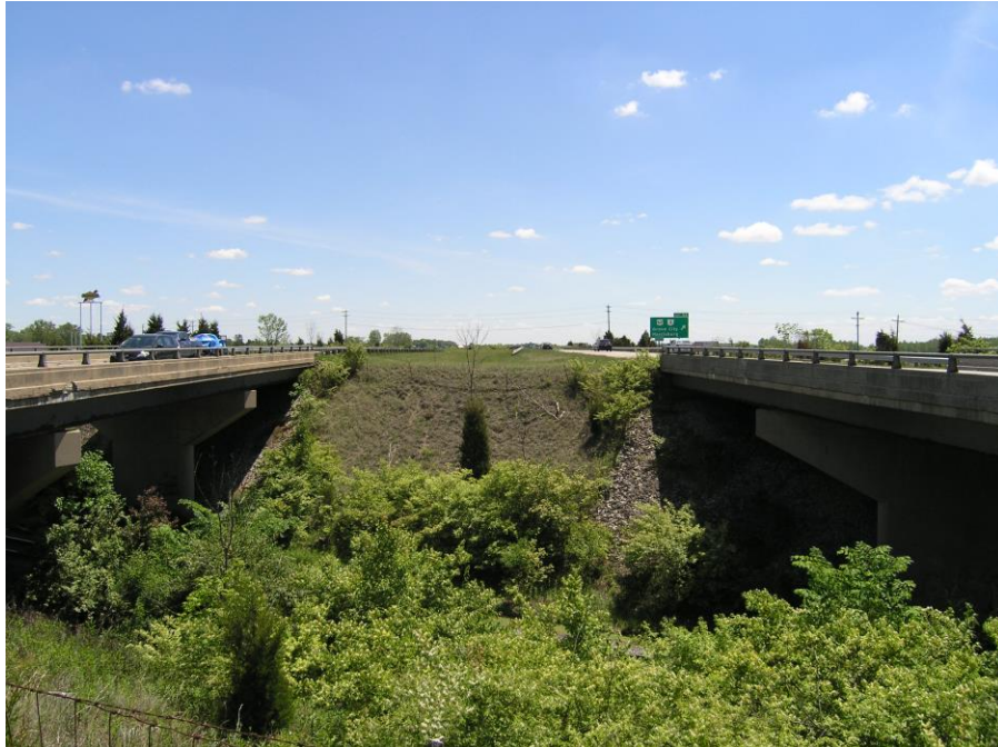
Photograph 4: Looking North from Rear Abutment – Area to be widened.
