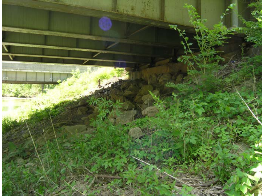
Photograph 3: Rear Abutment of SB Structure.
