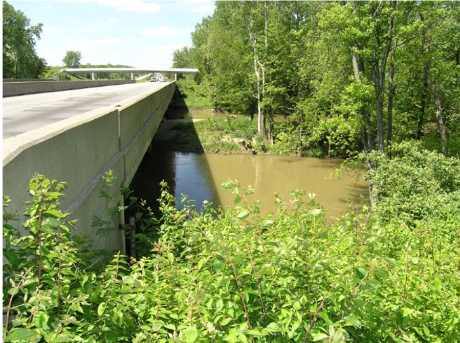
Photograph 4: Left Channel of BDC from SB Structure Looking South (west).
