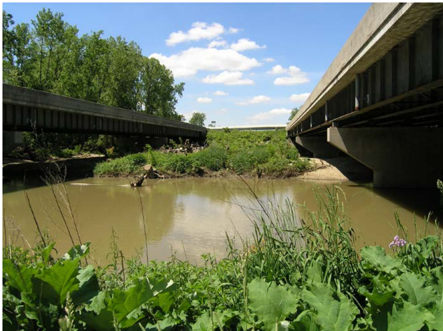
Photograph 5: Area to be Occupied by Widening
