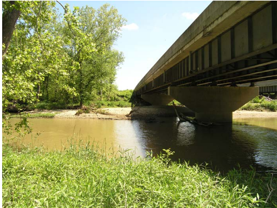
Note presence of island blocking much of the channel between Piers 1 and 2.
