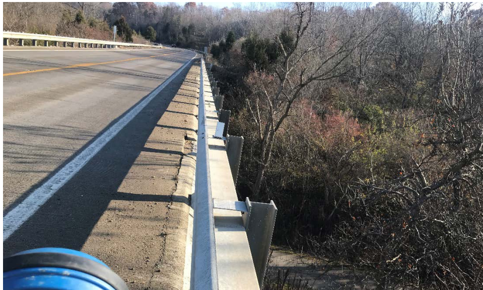
Photograph 4: Bridge Deck Wearing Course Surface
