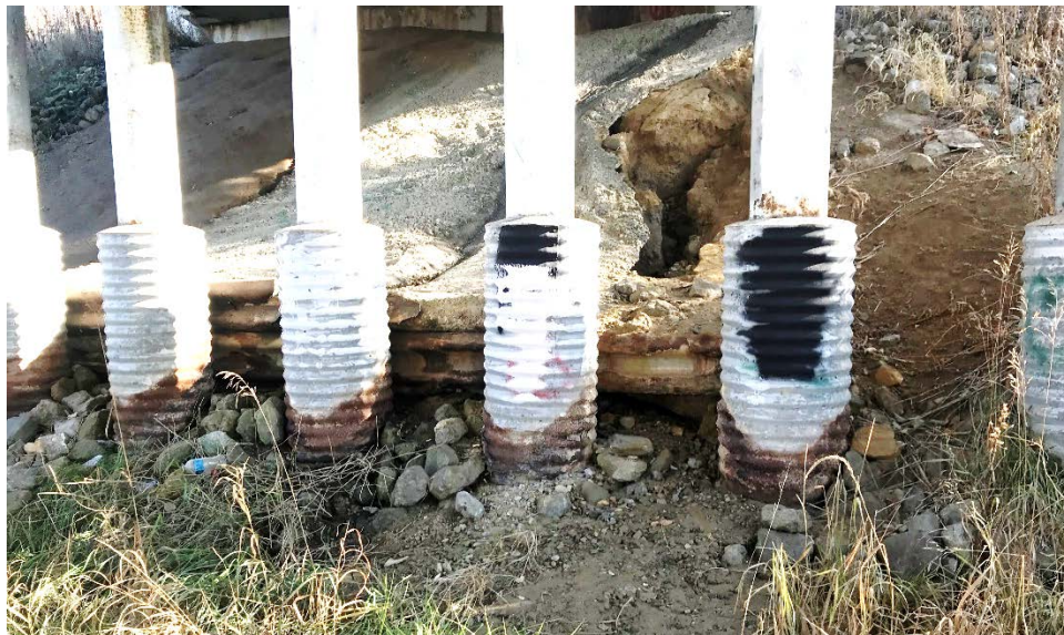
Photograph 2: Forward Abutment Slope
