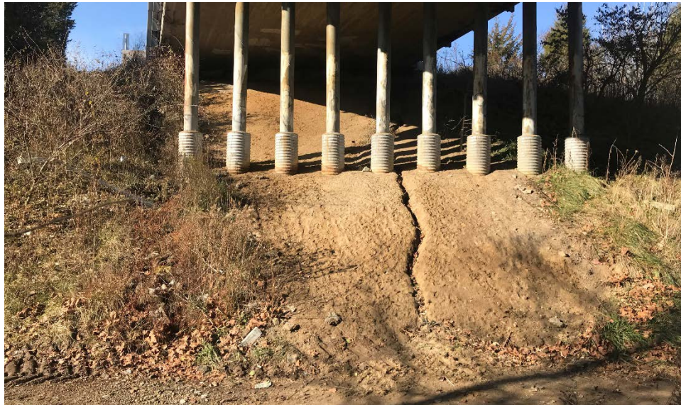
Photograph 1: Rear Abutment Slope
