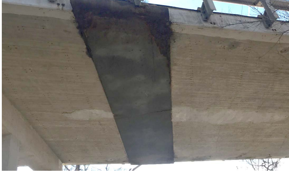
Photograph 3: Underside of Bridge Deck
