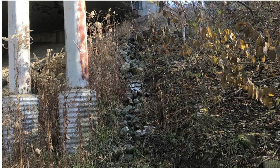
Photograph 5: Spill-Through Slope with Drainage Swale Protection
