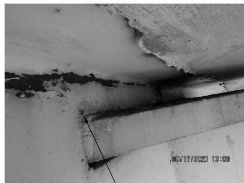
CRACKED WELDS
