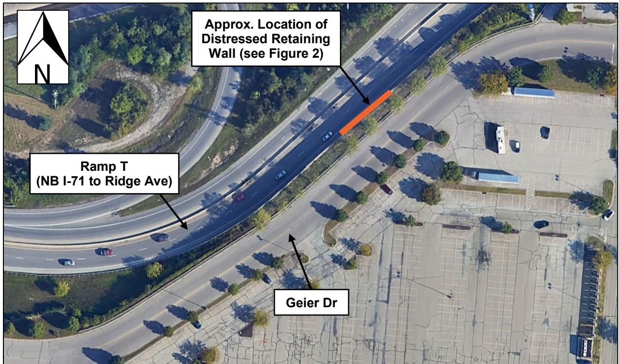
Figure 1: Site Vicinity (from Google Earth Pro, Imagery Date: 9/10/2023)
