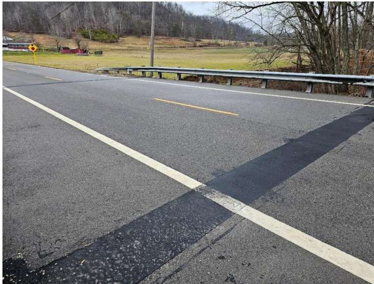
Photograph 4: Asphalt wearing course
