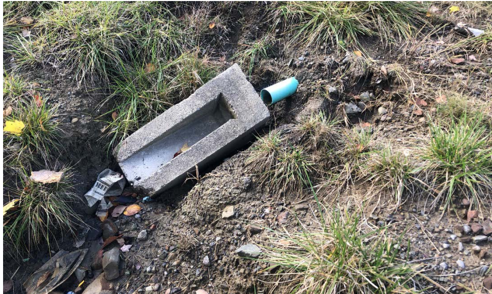
Photograph 4: Drainage Basin Outlet in Eastern Embankment
