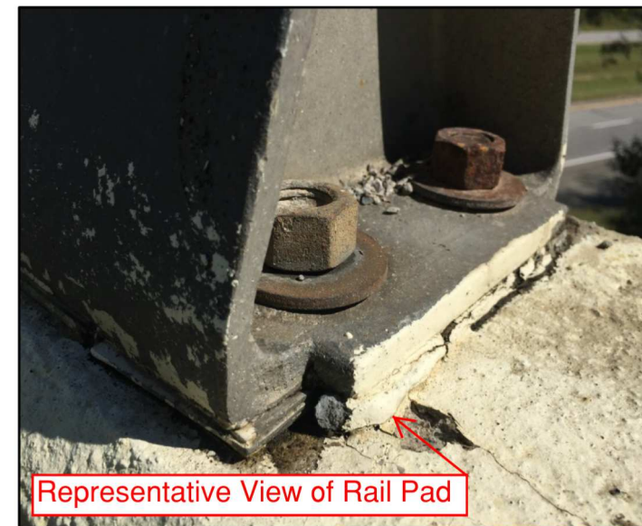
Representative View of Parapet Wall Caulking
