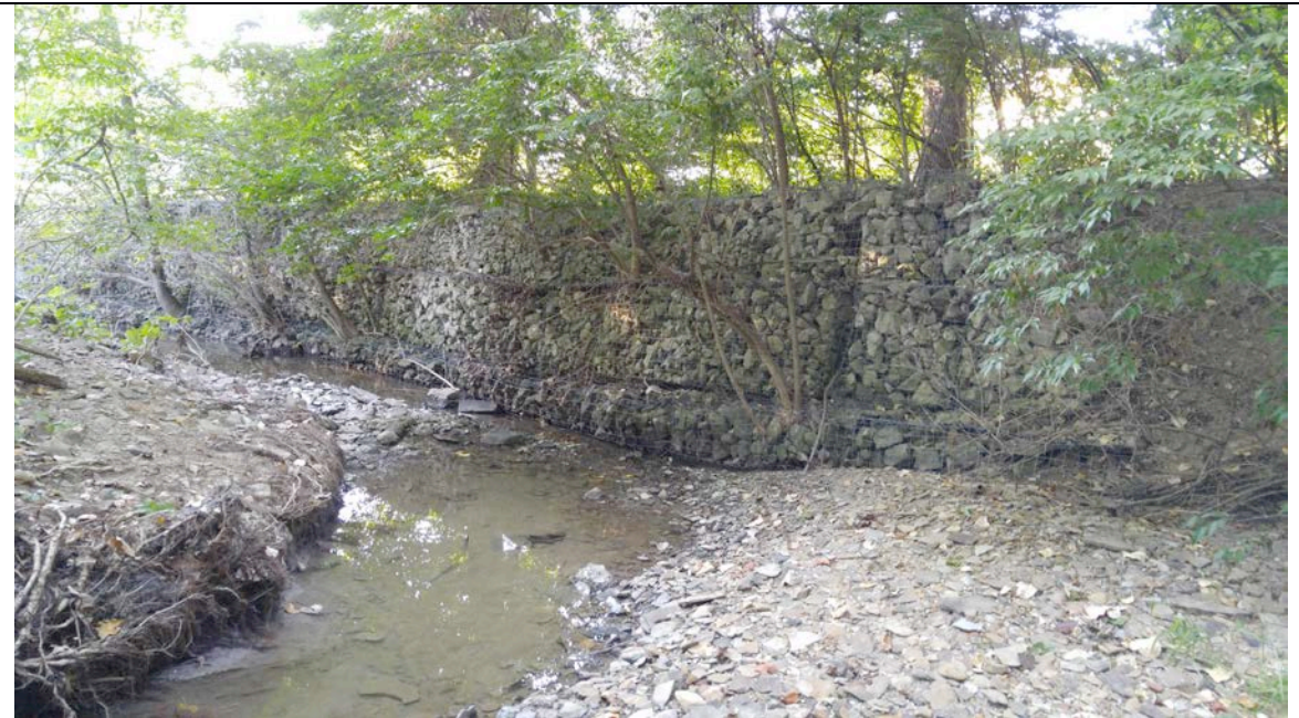
Photograph 38: Gabion wall at River Styx Rd culvert at Sta 900.
