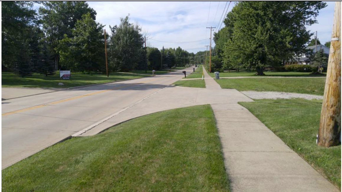
Photograph 30: Sidewalks along Foote Rd.
