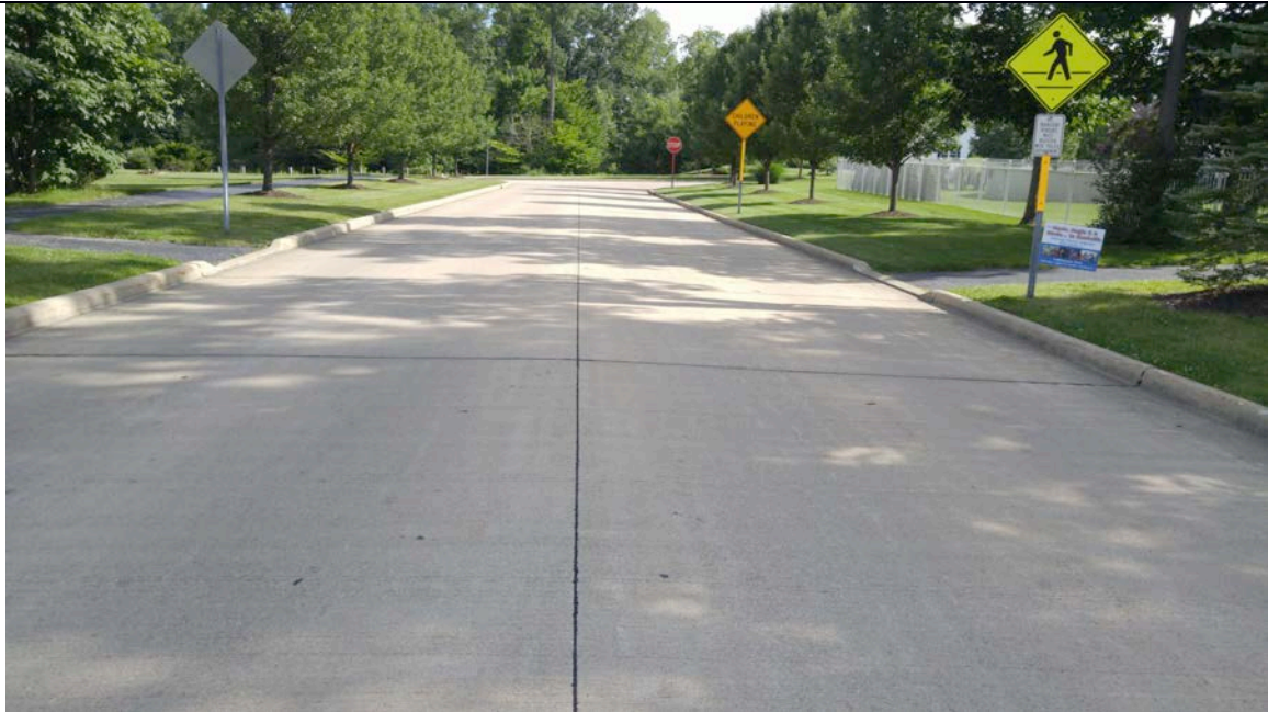
Photograph 28: View of concrete along Foote Rd and surrounding residences.
