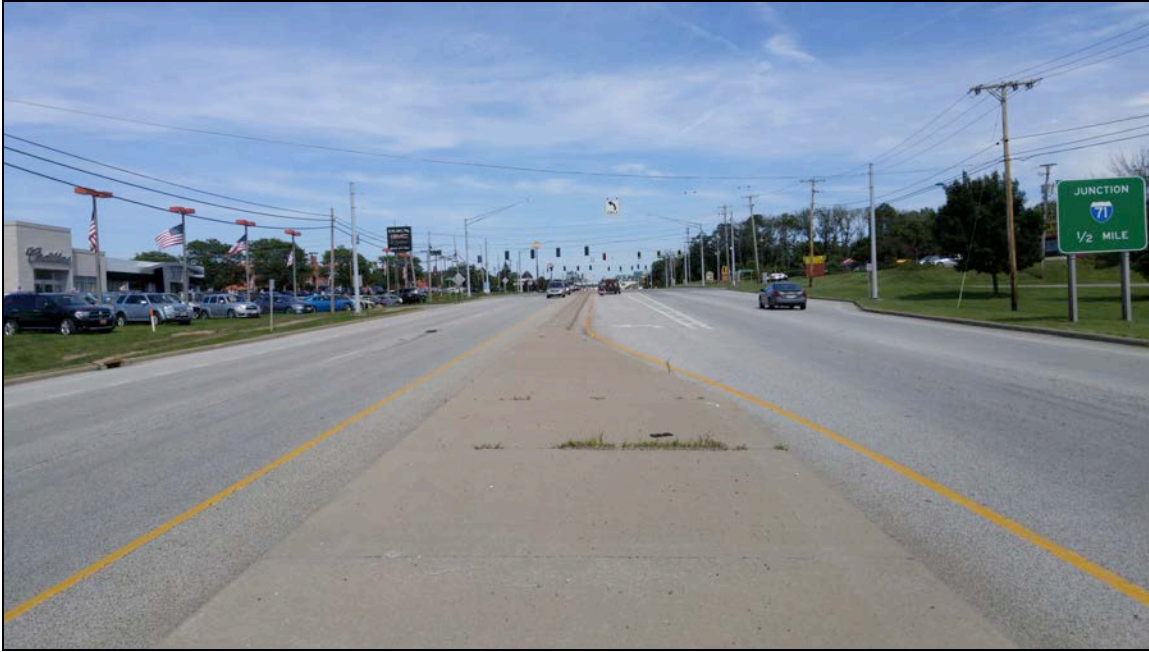
Photograph 1: SR-18 near Sta 193+00 where median changes to a curb.
