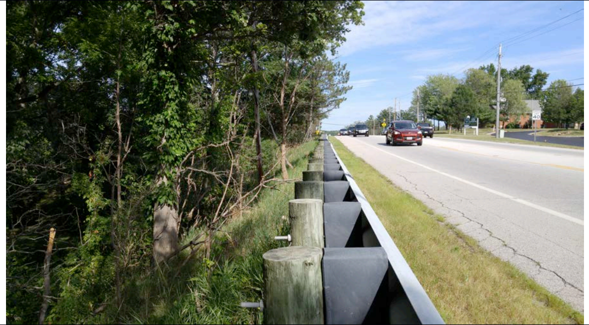
Photograph 17: Guardrail at historical landslide near Sta 127
