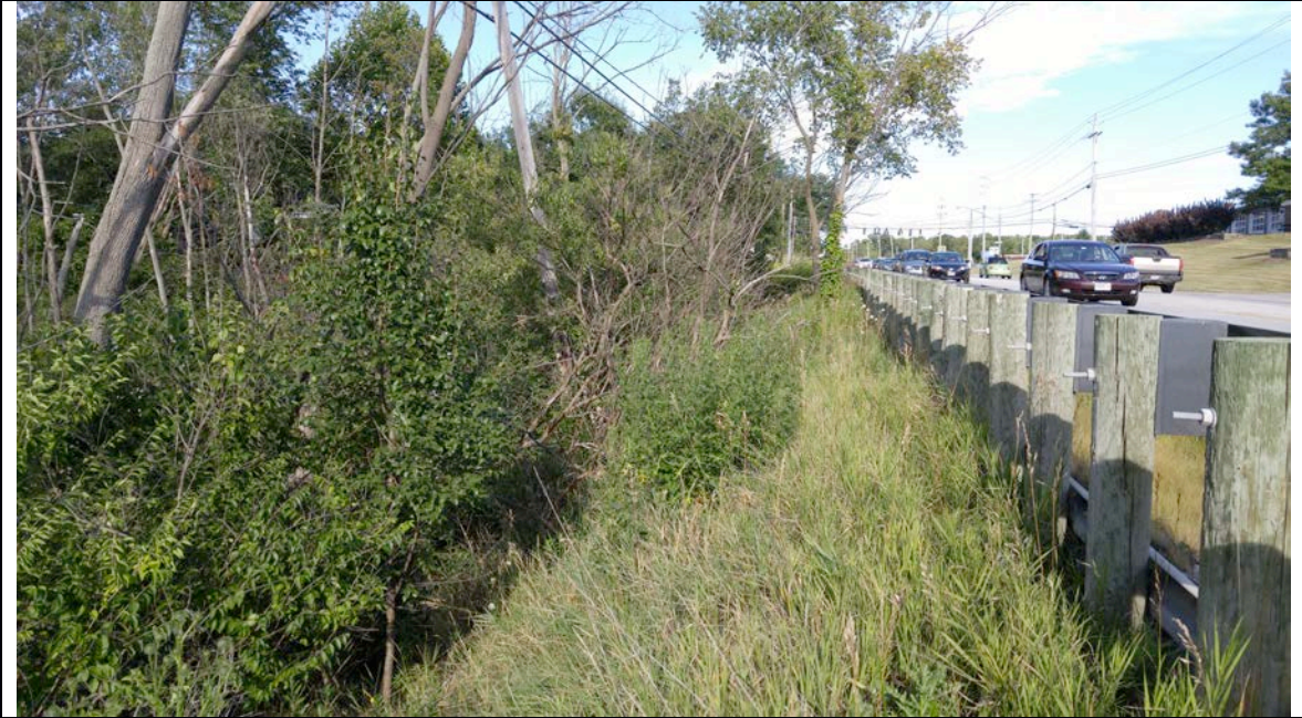
Photograph 21: Guardrail at historical landslide near Sta 166
