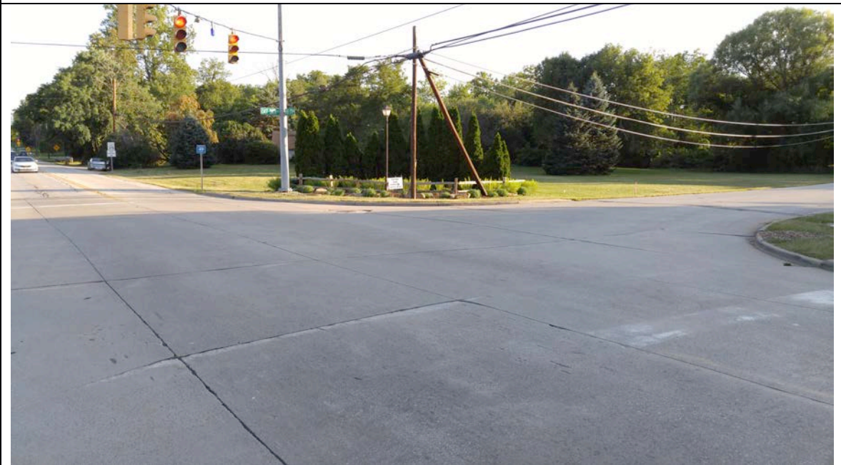
Photograph 36: River Styx Rd and E Smith Rd Intersection
