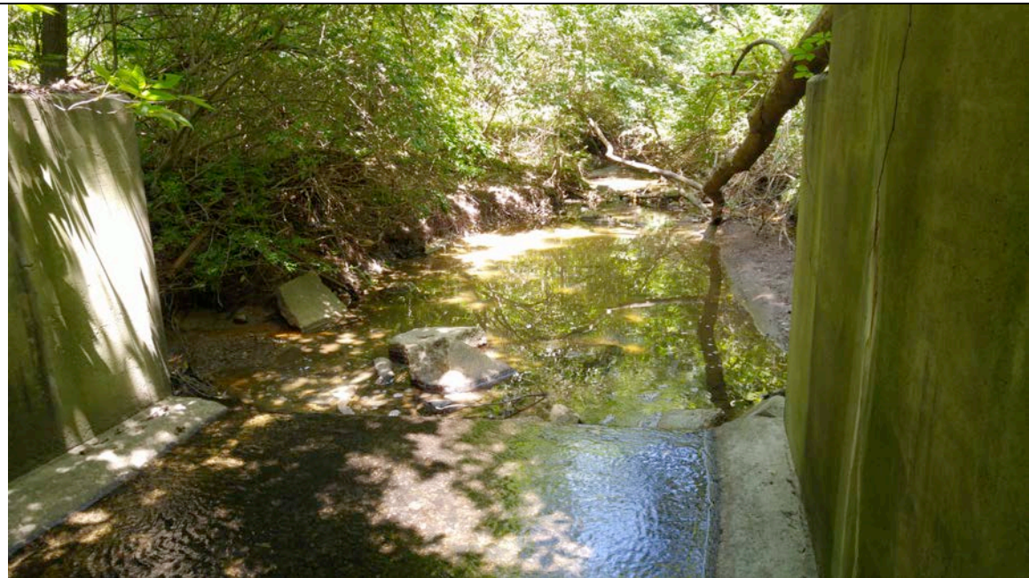
Photograph 4: View of Broadway Creek at SR-18 ~Sta 102+55.
