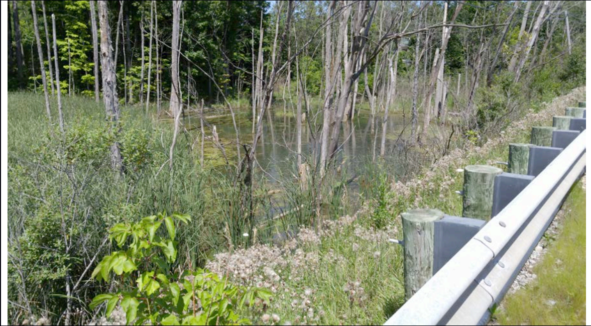
Photograph 19: Swamp at historical landslide near Sta 166
