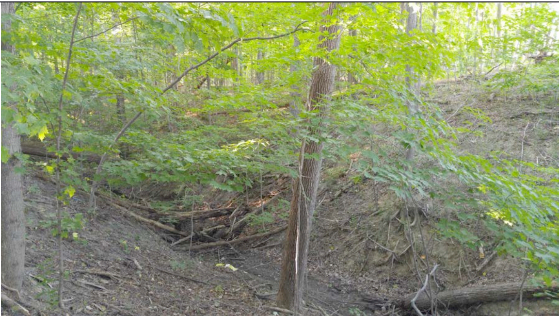
Photograph 26: Erosion along creek at the site of the northern Frontage Rd
