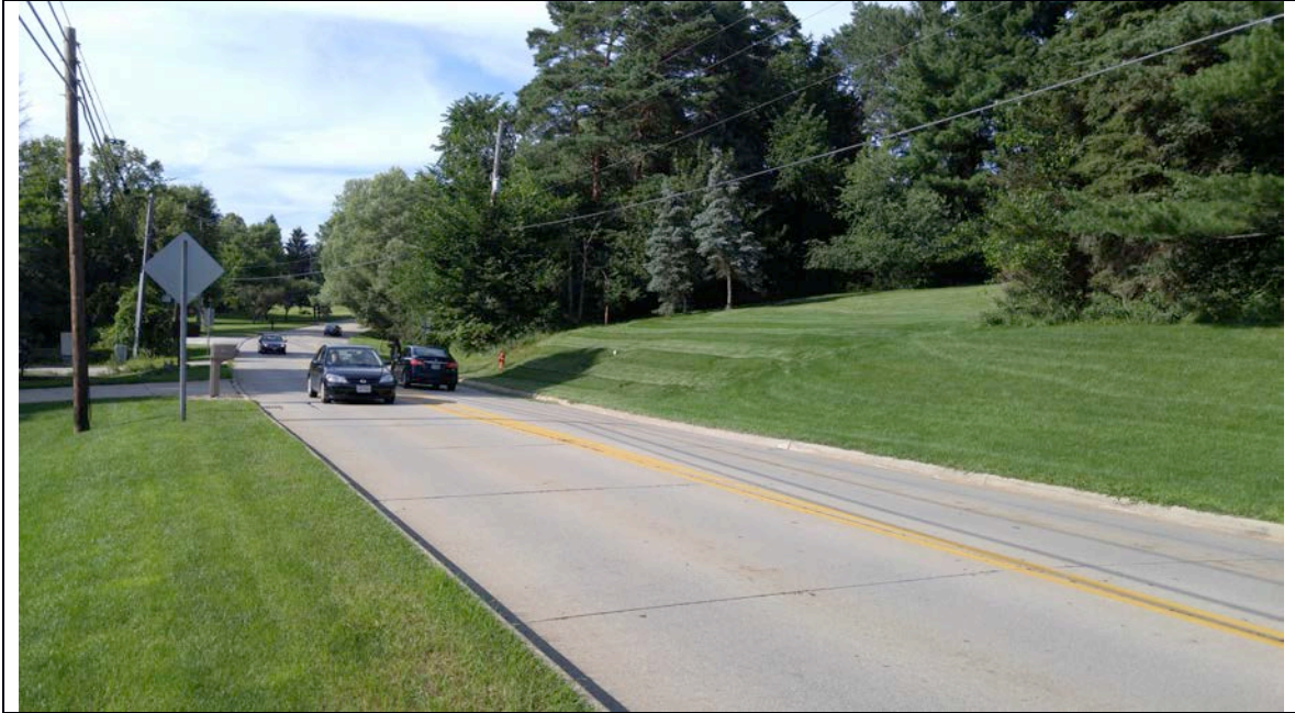
Photograph 31: View of the sloping terrain along the southern end of River Styx Rd.
