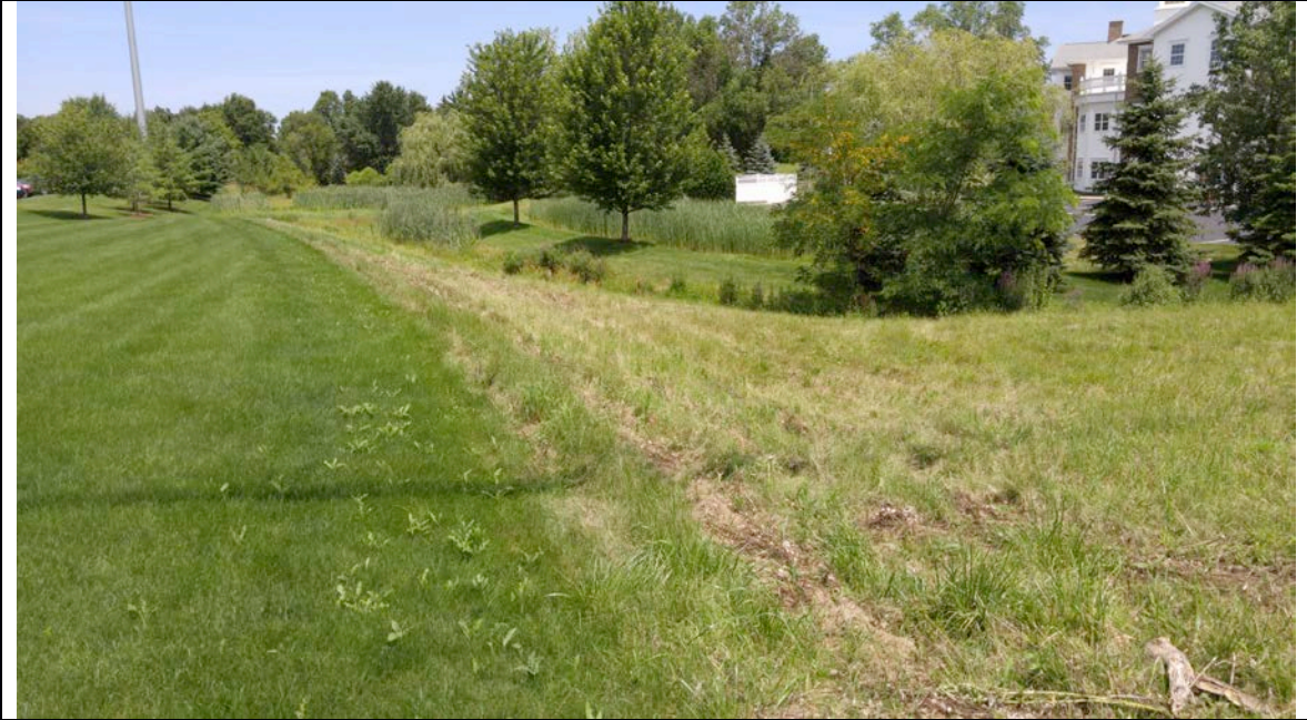
Photograph 13: View of a marsh north of SR-18 at ~Sta 111+50.
