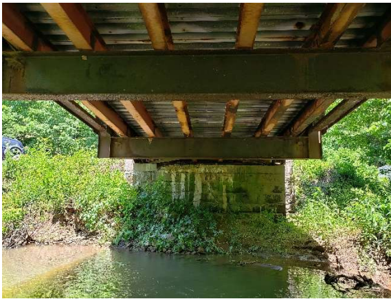
Facing North Abutment
