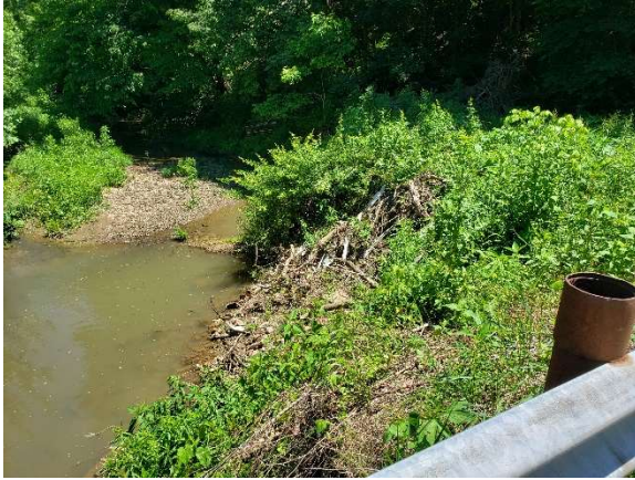
Bank Southeast of Bridge (Debris at Bend)
