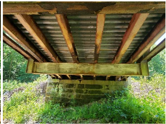
Facing South Abutment
